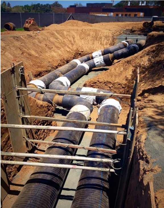
Figure 11 - Distribution System Conversion Example
