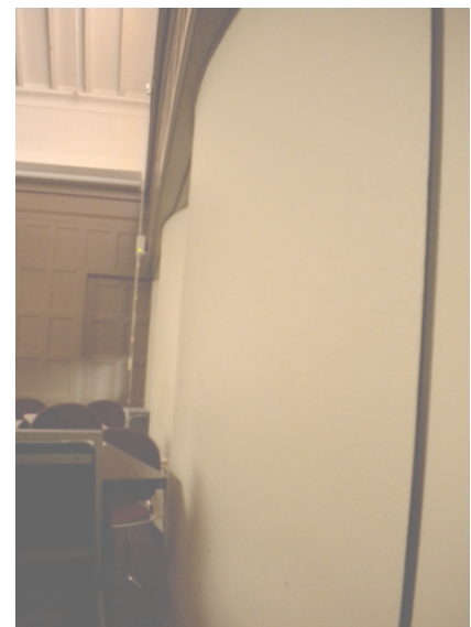
^ SOUTH WALL - ACOUSTICAL PANELS.
