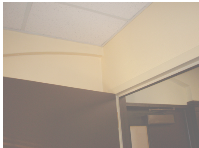
^ ENTRY ARCHWAY DETAIL.
