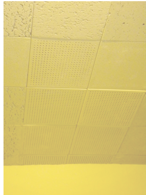
^ SOUTH HALLWAY CEILING DETAIL.
