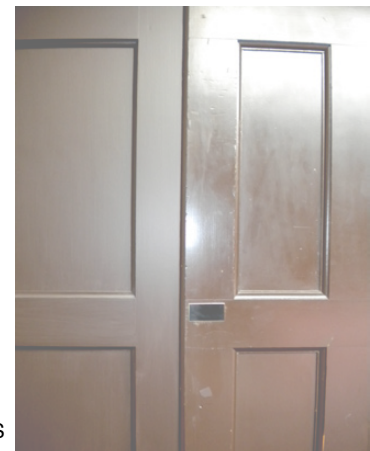
EXAMPLE OF DIFFERENT FINISHES (NEW VS ORIGINAL). >
