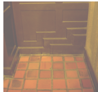
^ STAIR BASEBOARD AND TILE DETAIL.
