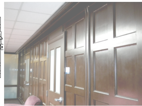
^ WALL DETAIL - NEW PANELING.
