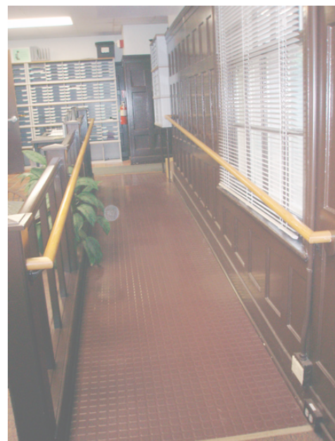
^ NEW RAMP AND WALL PANELS.
