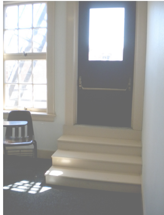
^ NORTH HALLWAY 3RD FLOOR FIRE ESCAPE.
