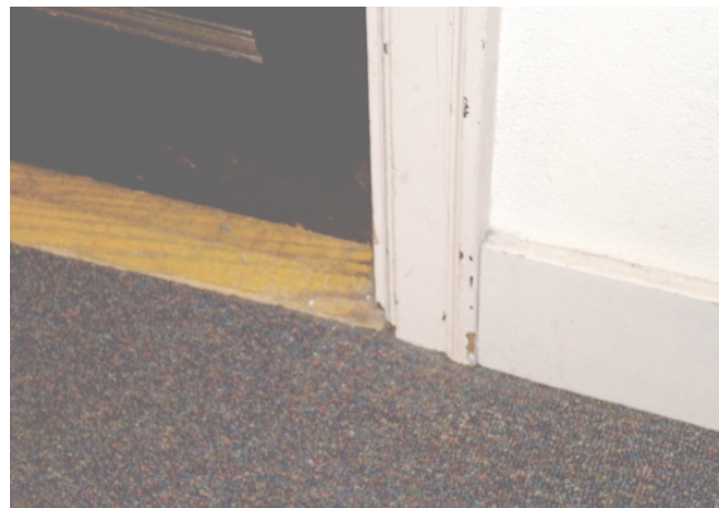
^ SECOND FLOOR BASEBOARD DETAIL.
