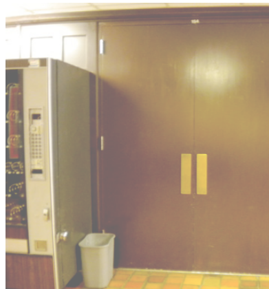
^ ROOM 154 - New (UNUSED) DOORS.
