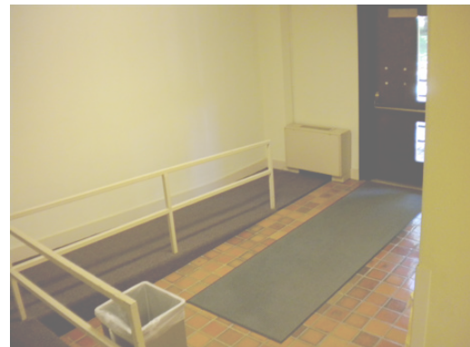
^ SOUTH HALLWAY ACCESS RAMP.
