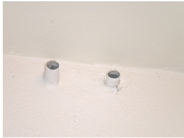
^ NORTH HALLWAY PIPE CUT OFF.
