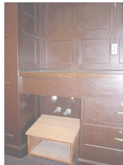
^ FORMER SINK STATION.
