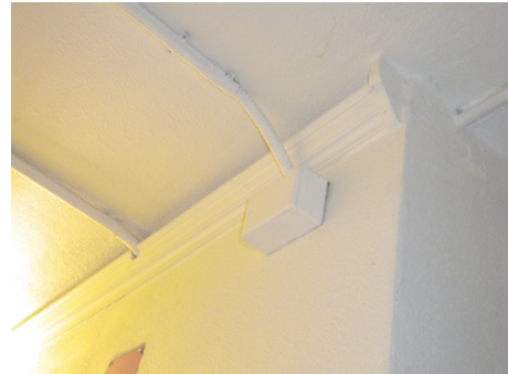
^ SOUTH HALLWAY MOLDING DETAIL.
