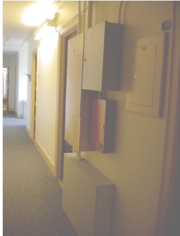
^ SOUTH HALLWAY THIRD FLOOR.
