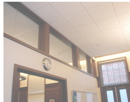
^ NEW PARTITION WALL.
