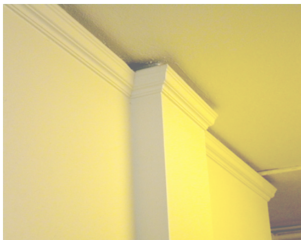
^ MOULDING DROP DETAIL.
