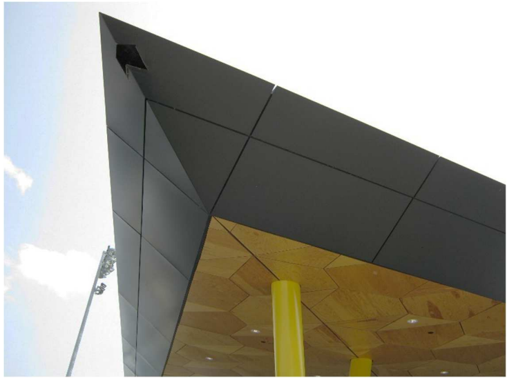
Figure 2: Roof Drain into Planter 1
