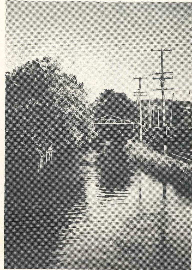
THIS WAS THE MILLRACE as it last looked—and as it will never look again. The photo was taken about 1940 from the Anchorage looking up stream. The wooden bleachers on the right were seats for the crowds who watched the annual canoe fetes. This part of the 'race was filled in, however, to make way for highway relocation. A new channel was cut several feet north (left) of this area.
