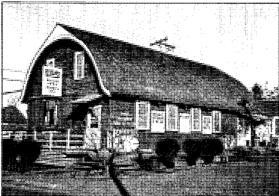
The Blair Boulevard Historic Commercial Area is working class district characterized by a mix of building types that are located along a diagonal boulevard with a quantity of large shade tree.
