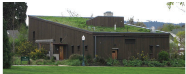
Many Nations Longhouse bioswale and green roof
