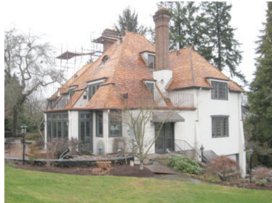
McMorrان House, East Elevation, 2009
