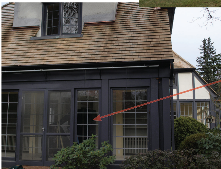
2009 - West facade showing enclosed living porch (date unknown).
