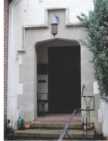
McMorran House, North Entry, 2009
