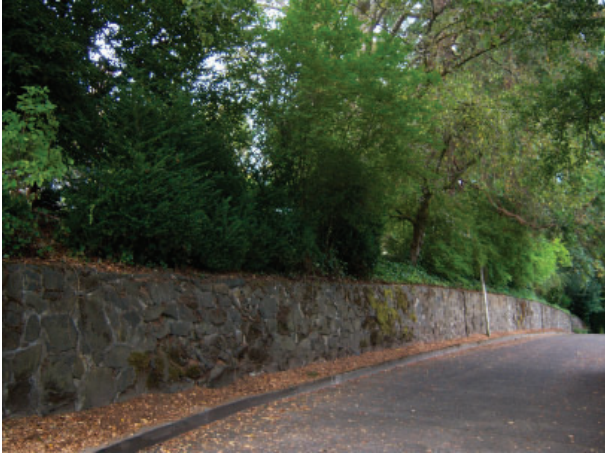
Exterior Basalt Wall (2009)
