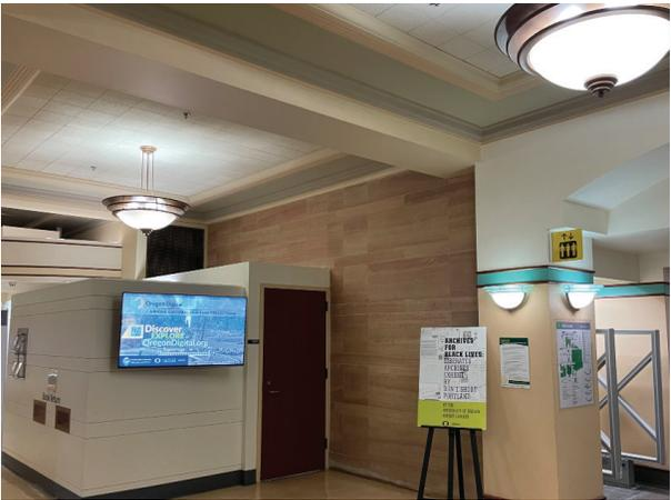
(2023) 1st Floor Lobby and Circulation Desk. Note the alterations to the south wall and reconfiguration of the circulation desk and lobby space (c1990). The kasota stone, ceiling and volume remain - further research needed to explore the ceiling configuration behind the altered wall.
