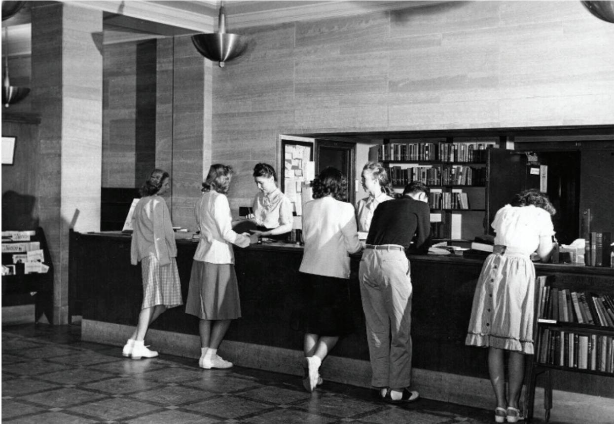
(c1950) 1st Floor Lobby and Circulation Desk. Note the original south wall, the wall opening/entry to the special collections behind the circulation desk, the original kasota stone walls, and ceiling and volume of the lobby.
