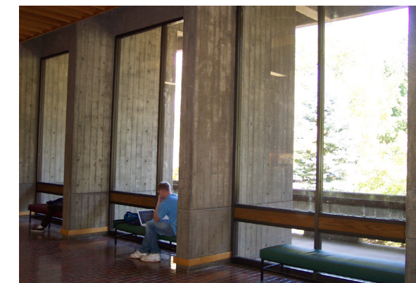
McKenzie interior showing roughcast concrete.
