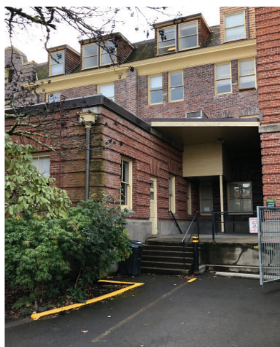
Dormers added to east facade. Overhang above the stairs and entrance is not original.
