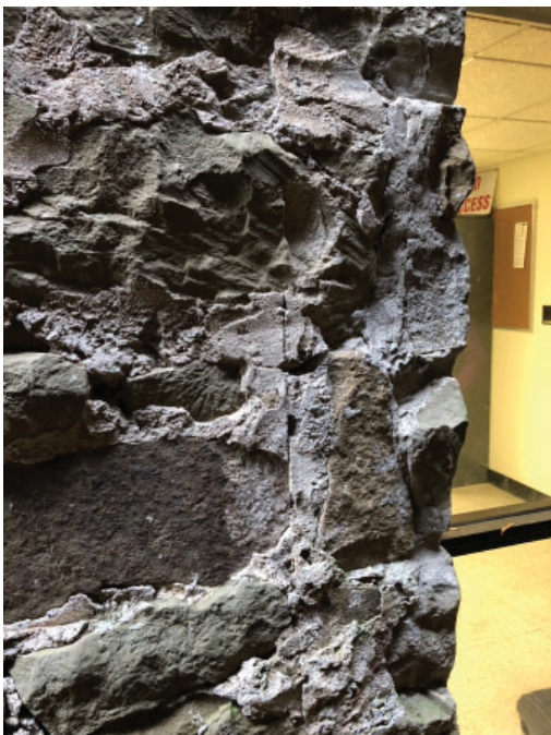
Original stone foundation throughout basement level.
