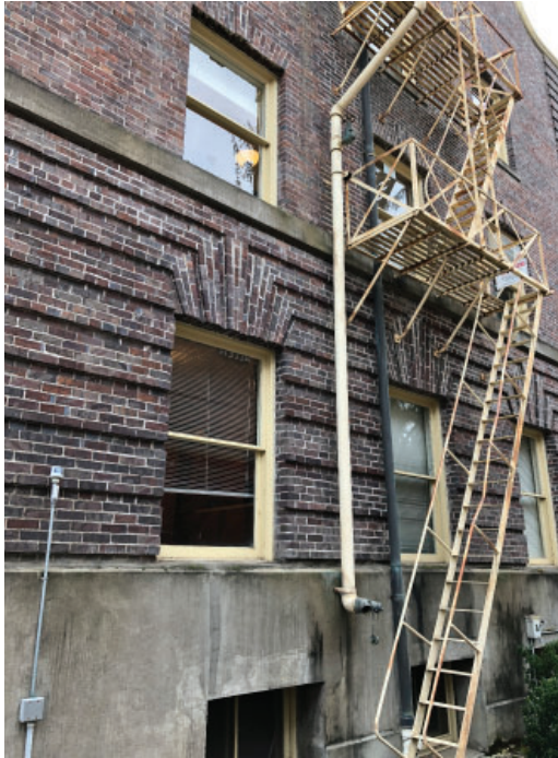
Fire escapes are not original, further research needed to determine date added. Fire sprinkler standpipes are not original.
