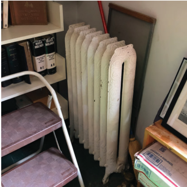
Room 323 (Ornamented Radiator)
