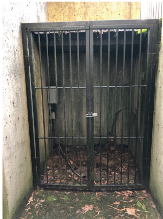
Gated storage on west facade below grade is not original.
