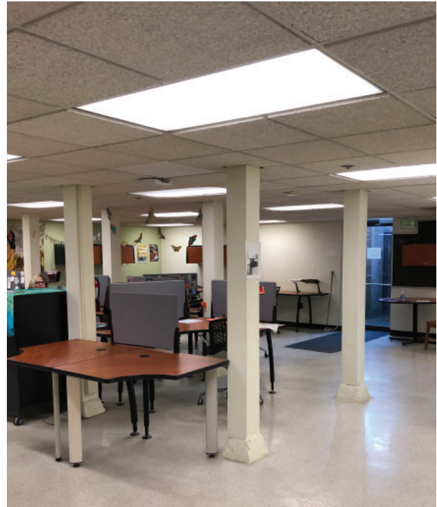
Support pillars not original; further research needed for year pillars were placed/replaced
