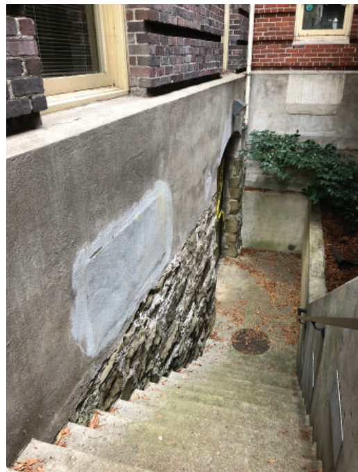
Difference between original stone foundation and 1914 addition foundation. 1914 addition used different colored brick
