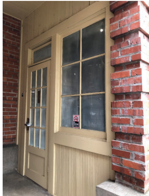
Original doors and windows.
