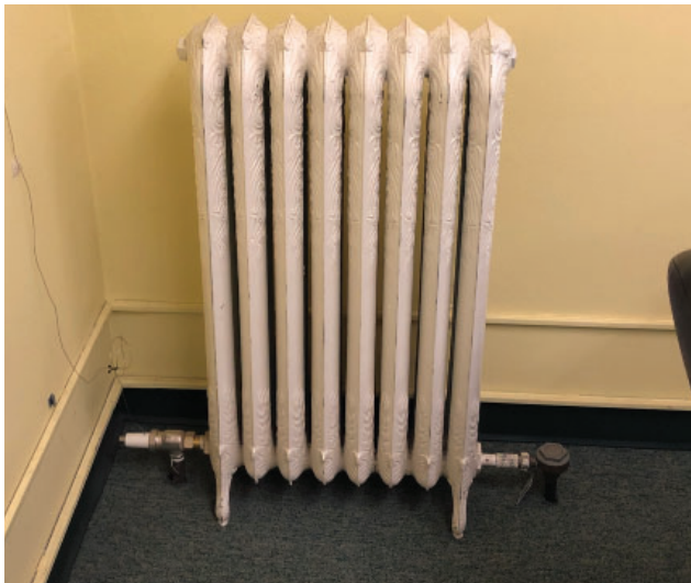
Room 308 (Ornamented Radiator)
