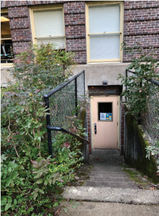
Light fixture above basement door is not original. Fenced stairwell is not original.
