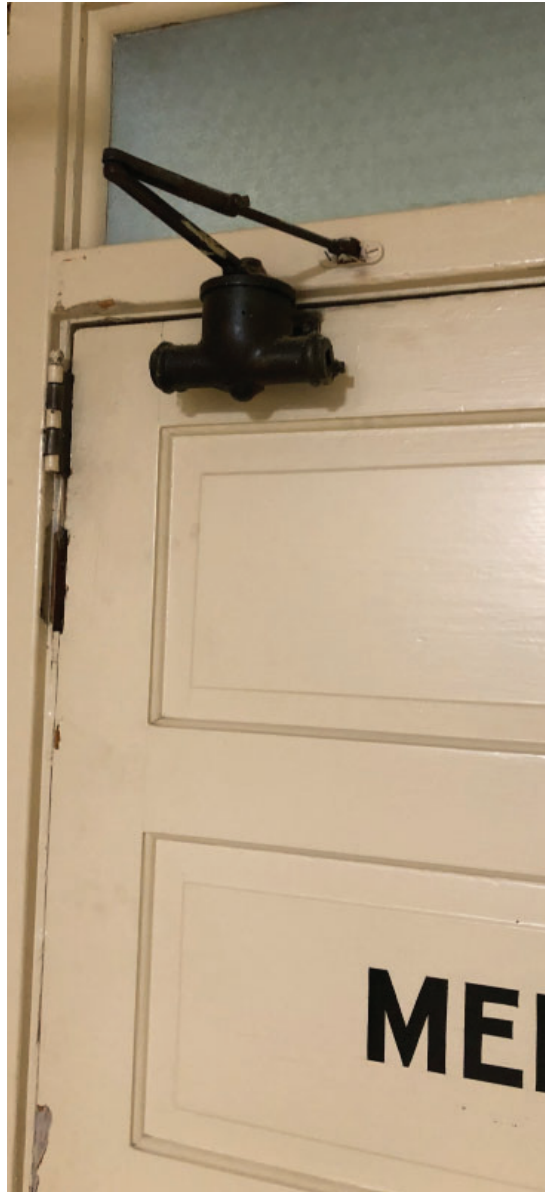
Mens Restroom (Old Hardware)
