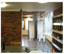
One of three openings in lobby cut in original exterior wall to make way for 1973 skybridge.
