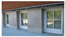
(3) Three sets of double doors replaced by double-over-double windows in 1985.
