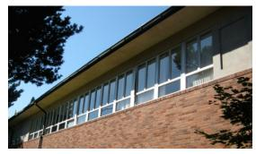
East-facing office windows replaced in 2009, with original stone panels (top right)
