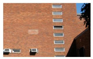
Infilled window on second floor at the time of 1985 addition of ballroom backstage.
