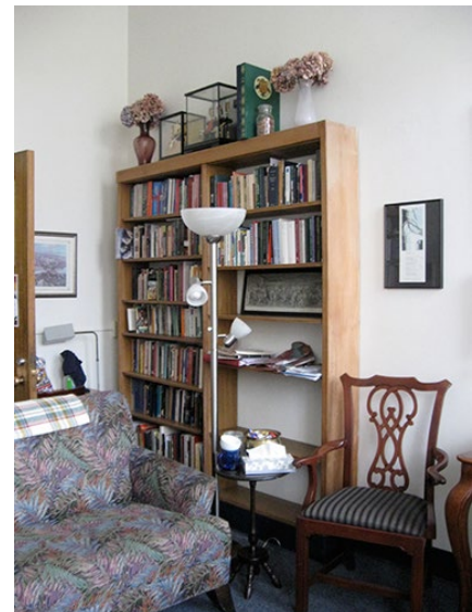
Original built-in bookcase in Room 212. The cabinet along the south wall and two sections of the bookcase indicated in the original 1938 drawings are no longer existing. March 2015.
