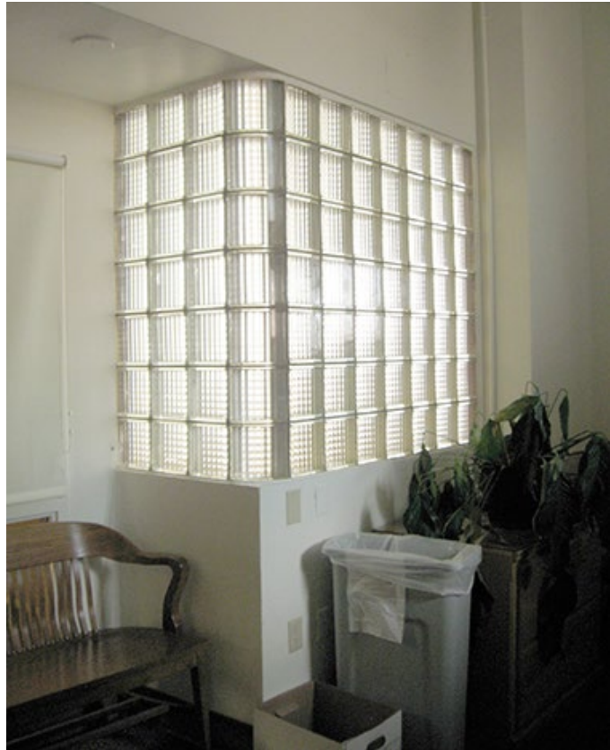
Original glass block wall in Room 320. March 2015.
