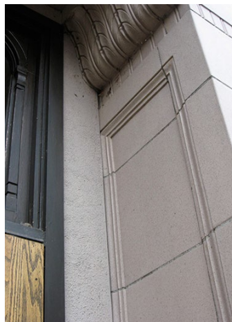
Existing original terracotta detailing, with concrete wall framing the relocated door. 2011.
