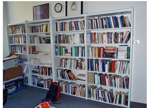
Built-in bookcase. Original drawings indicate 5 sections instead of the 4 in this photograph. 2011.
