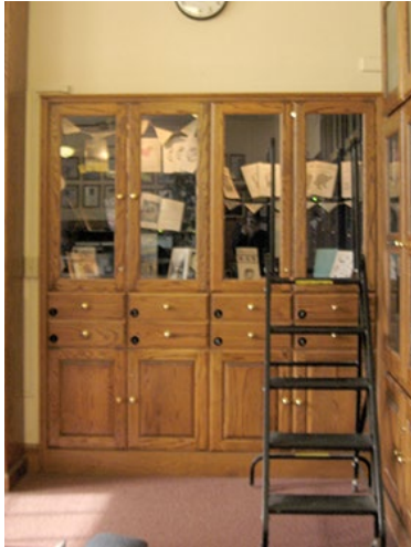
Built-in cabinet on west wall. Configuration matches original drawings but it is presumed that the cabinet faces have been replaced. March 2015.
