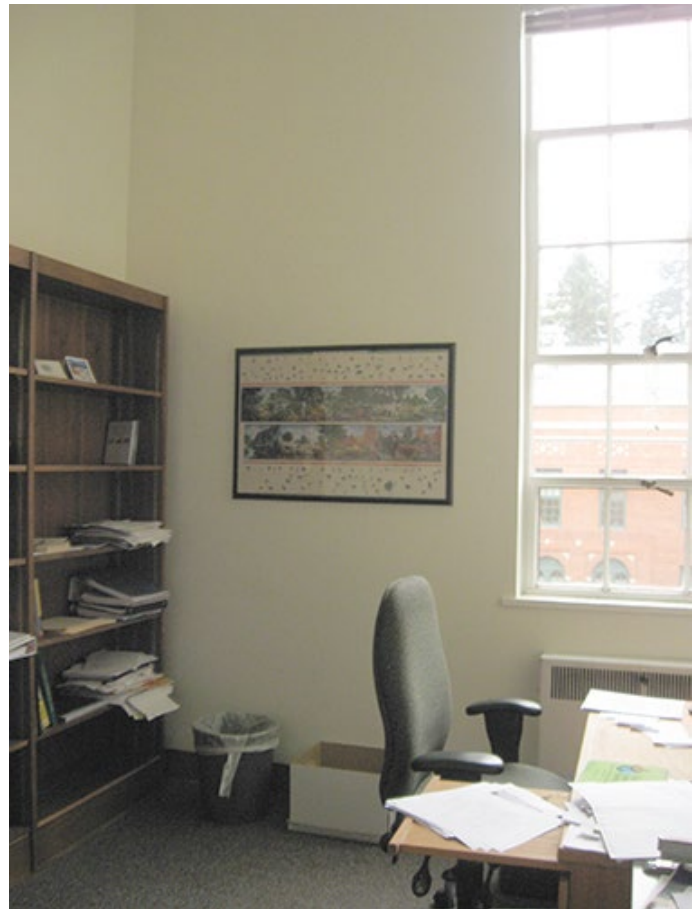
View of northwest corner of Room 320B. Notice placement of built-in bookcase compared to the original drawings above. Also note the difference in construction compared to the original bookcase in Room 320A seen in the photo above. March 2015.
