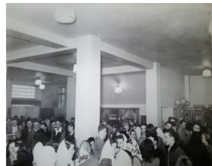
Cooperative Store with original plastered ceiling roughly 12' high, & original light fixtures. 1945.
