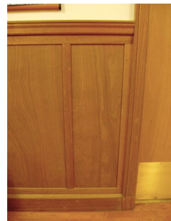
Detail of third floor corridor finishes. March 2015.
