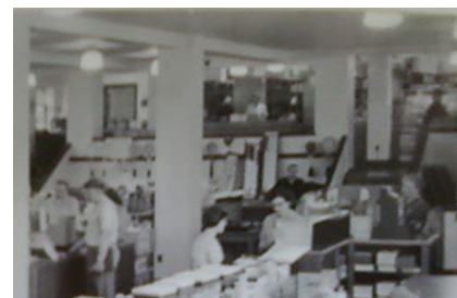
Store showing original configuration with two sets of stairs to first floor mezzanine in rear, with partial walls. 1945.
