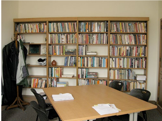
Original built-in bookcase in Room 320A. Currently about 1 foot shorter than indicated in original Ellis Lawrence drawings. March 2015.
