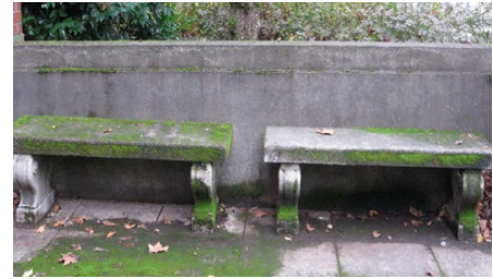
Original cast stone benches & 2' tiled concrete slab (west side). 2011.
