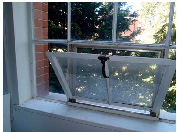
Steel frame hopper window opening. 2011.
