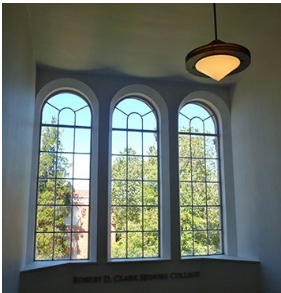
Original arched windows and original decorative pendant light. 2011.
