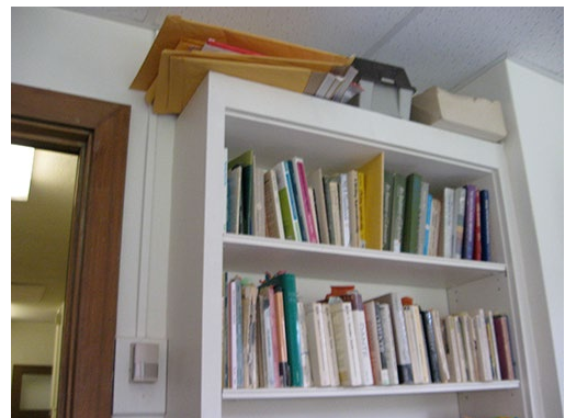
Built-in bookcase in location of original built-in bookcase. Shelves appear to be original, but painted. Trim around the case appears to have been altered. March 2015.
