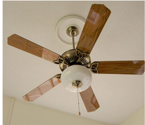
Existing lighting in Room 320A and 320B. March 2015.
