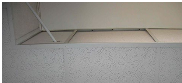
1966 dropped ceiling w/ perimeter soffit exposing original plastered ceiling above.
