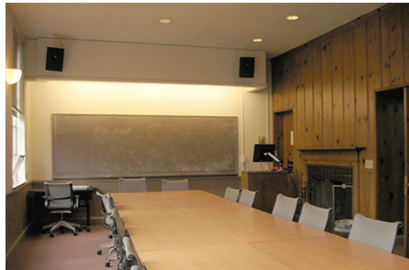
Existing conditions of Room 303, looking west. March 2015.
