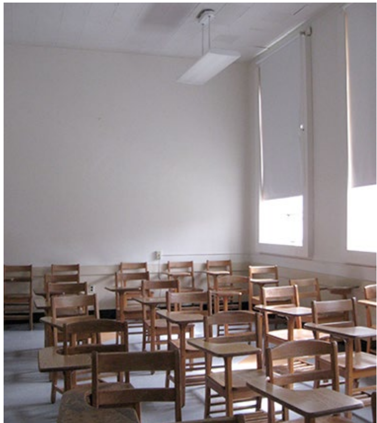
Southeastern corner of Room 204. March 2015.
