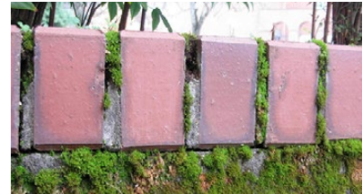
Detail of original 45° edge-cut of brick cap on concrete retaining wall. 2011.
