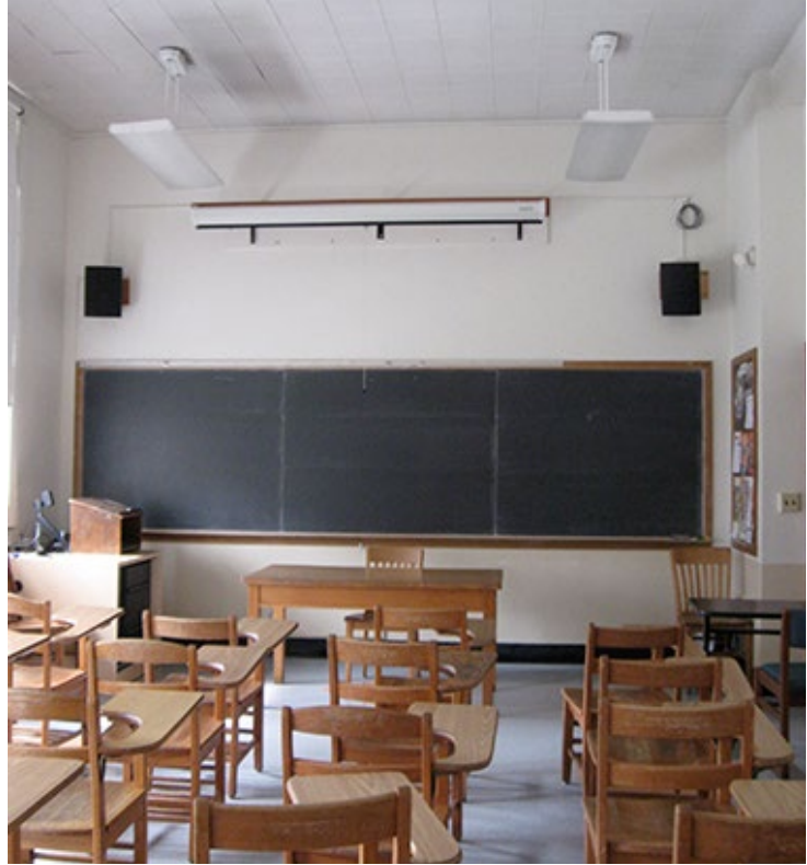
Western interior wall of Room 204. March 2015.
