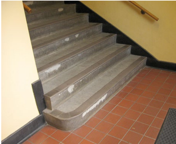
Detail of stairs from Main Entry. March 2015.
