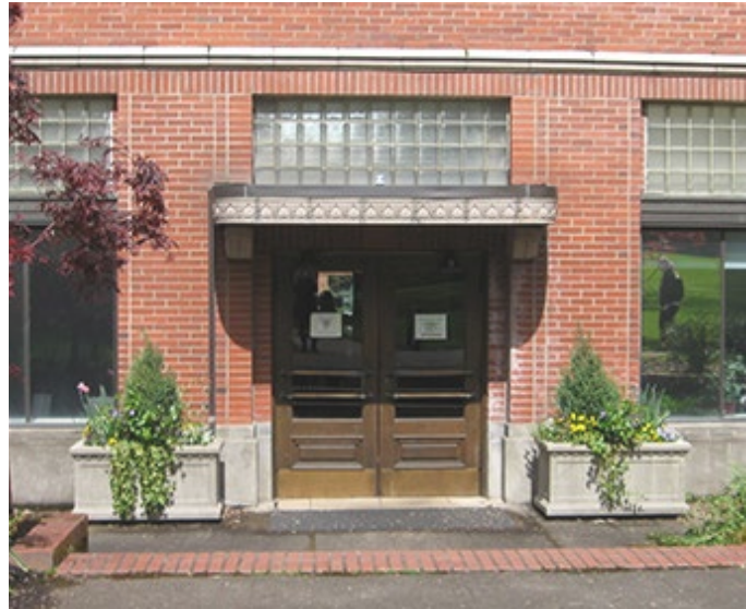
South Entry with original door and hardware and new awning April 2015.
