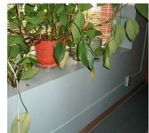
Original concrete window seat in bay windows. 2011.
