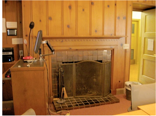
Original fireplace with wood mantel and knotty pine paneling. March 2015.
