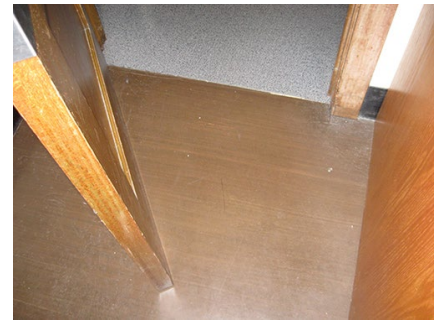
Original jasje linoleum flooring in Room 222. March 2015.
