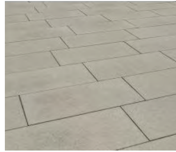
3: Cast in place concrete - Uniform finish Pedestrian scale paving pattern, simplified variance of mixing zone Color change in parking areas
