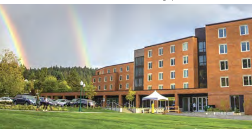
Photo: Kalapuya Ilihi Residence Hall.
