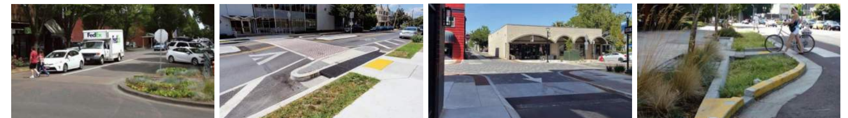
Curb extension or bulbout
