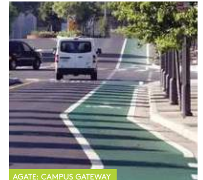
AGATE: CAMPUS GATEWAY A CAMPUS CONNECTOR AND GATEWAY, WITH BIKE LANES AND SAFE CROSSINGS FOR PEDESTRIANS
