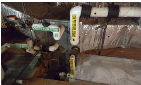
Typical Duct Mounted Heating and Cooling Coil
