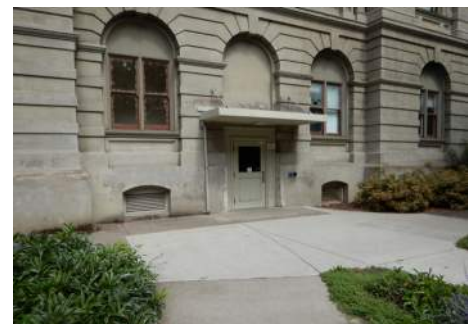
Existing Accessible Entrance at South Elevation
