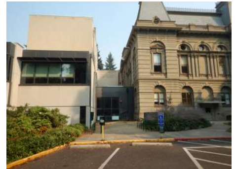
Existing Accessible Parking at South Elevation
