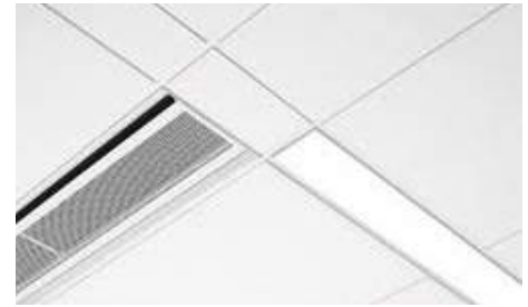
Install chilled beam
