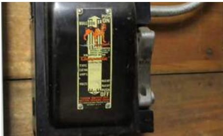
Example of a 67-year-old disconnect; typical throughout the building
