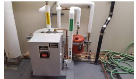
Typical Theater Electric Water Heater
