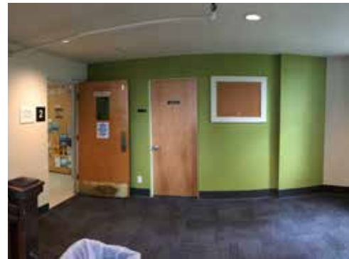
Image 56: Existing stair landings are enclosed by the use of offices, identified by the green wall in this image.
