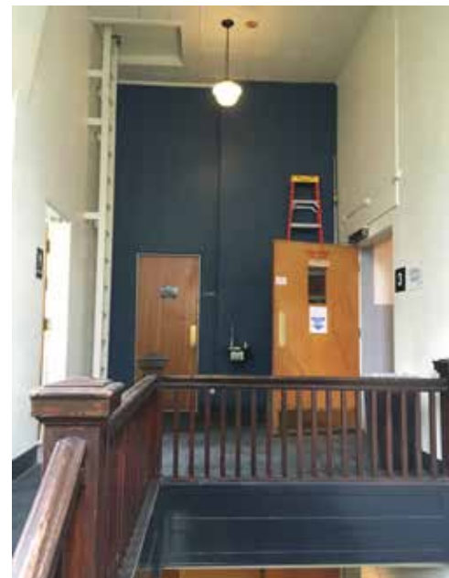
Image 58: The third floor stair landing is enclosed by an office (identified by the blue wall) and a restroom (door pictured left). The full-height windows within these spaces no longer provide natural light to the stairs.
