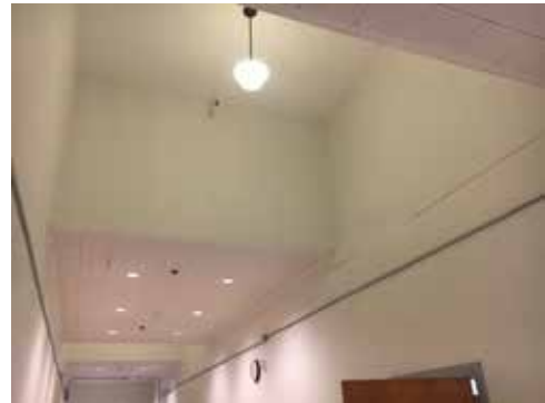
IMAGE E12: A mix of “schoolhouse” style pendant lights and recessed downlighting in a typical corridor.
