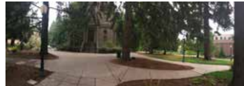
Image 73: Exterior sidewalks in good condition, with some cracking and upheaving from nearby tree roots.
