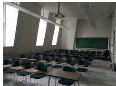
Image 6: A typical third floor classroom volume with tall ceilings and full-height dormer windows.
