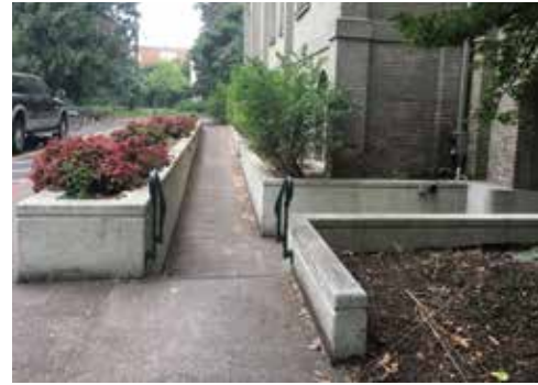
Image 72: Exterior ADA ramp at the north elevation, in fair condition.
