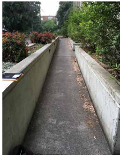
Image 46: Looking east up the concrete ADA ramp at the north elevation from the basement level landing.
