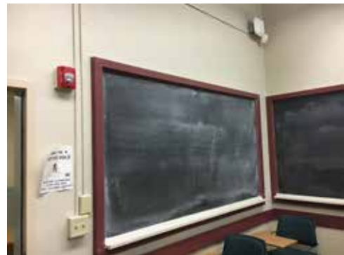
IMAGE E9: Surface conduit supplies power, data, and wifi outlets.
