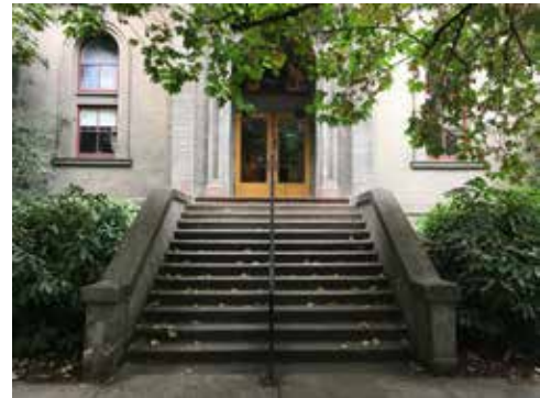
Image 2: The grand west elevation entrance with prominent concrete stairs.
