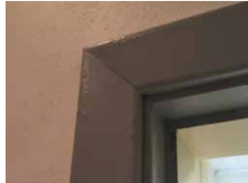
Image 68: Detail of typical interior door trim.
