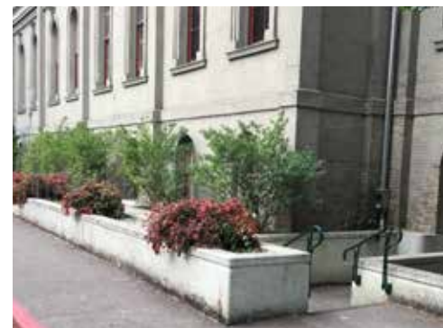
Image 43: Exterior view of the 1988 ADA ramp from the northwest corner of the project site.
