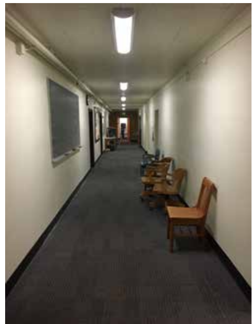
Image 49: The unwelcoming basement corridor, which serves as a primary corridor for those entering the building from the ADA entrance at the northwest corner.
