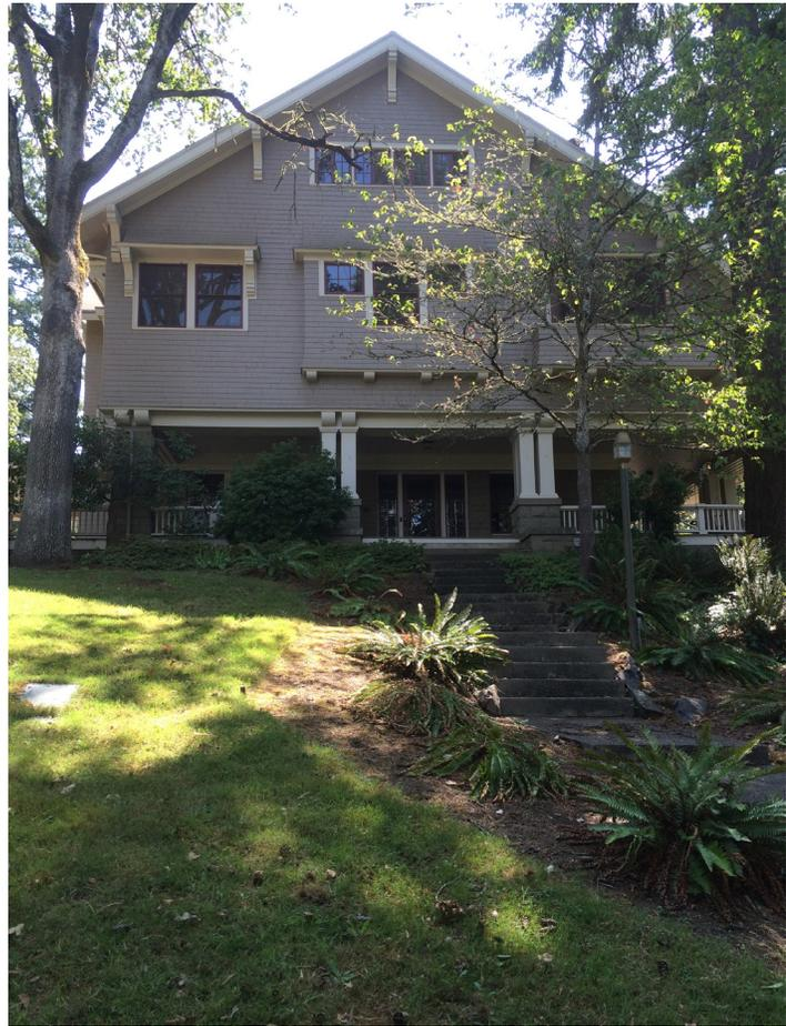
**Historic Materials:** Tenino stone-cut block foundation, columns, and facade; painted wood columns, corbels, eave brackets, and shingles; most likely the original 6/1 double-hung sash and sidelight windows.
