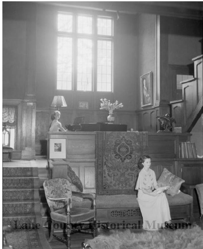
Historic Materials: dark stained oak beams; fireplace with bas-relief; wainscoting; casing; trim; built-in seating and cabinets; varnished, white oak flooring; brick fireplace and flooring; most likely the original 6/1 double-hung sash and sidelight windows.
