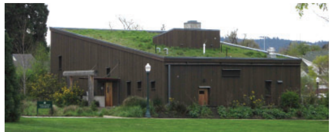
Many Nations Longhouse bioswale and green roof
