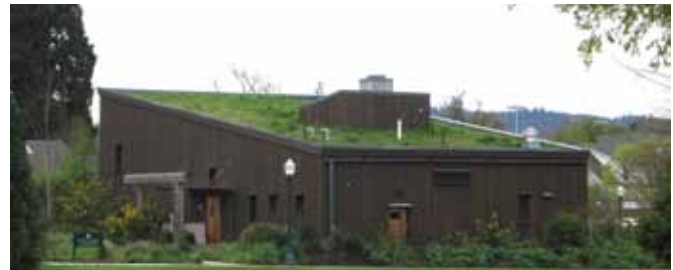
Many Nations Longhouse bioswale and green roof
