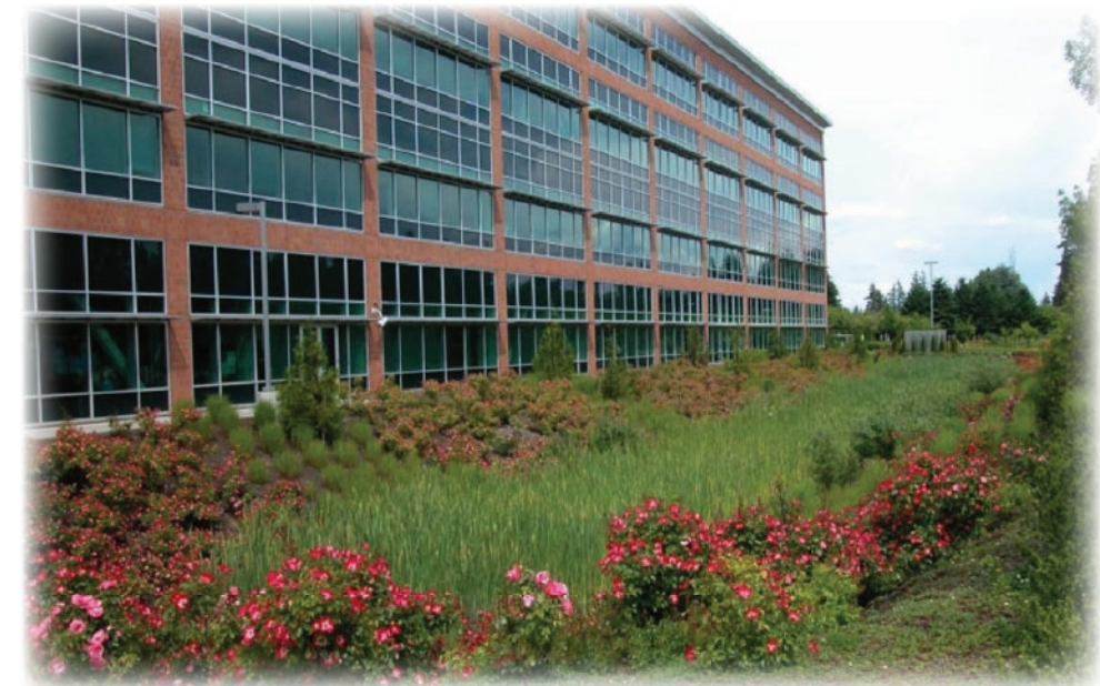
EXTENDED DRY BASIN- USED IN A PLACE WHERE YOU NEED TO TEMPORARILY DETAIN WATER RUN OFF DURING STORM EVENTS.
