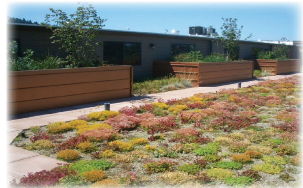
GREEN ROOF- USE ON SUITABLE ROOFS, GREAT TO REDUCE ENERGY COST, STORMWATER FEES, AND AESTHETICALLY PLEASING.
