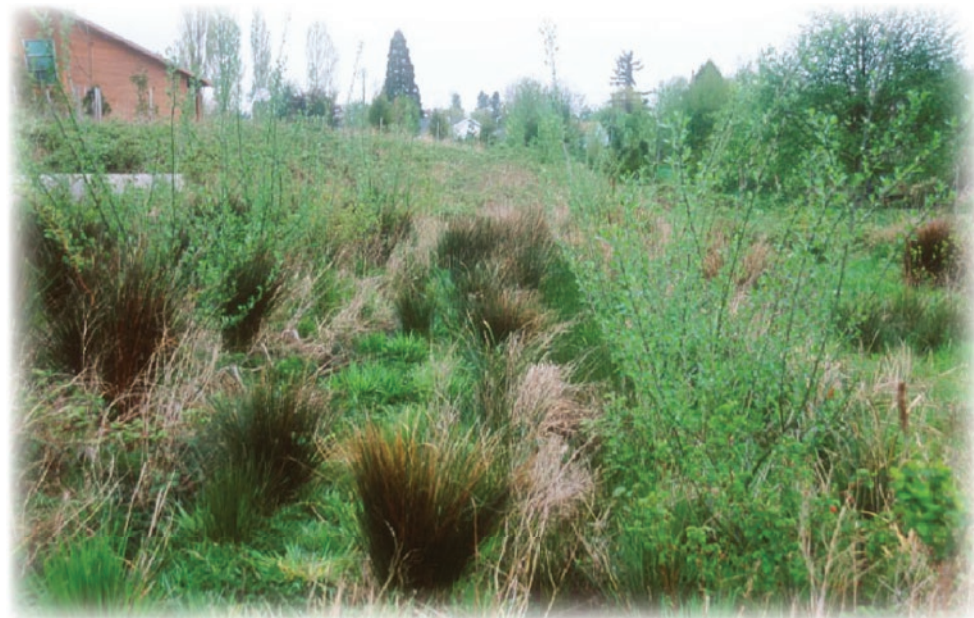
VEGETATED FILTER STRIP- USE WHEN ADJACENT TO IMPERMEABLE SURFACES SUCH AS PARKING LOTS, STREETS, ETC.
