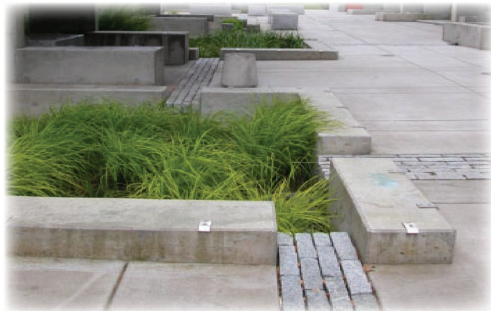
FLOW THROUGH PLANTER- USE IN AREAS WITH HARD SURFACES SUCH AS CURBS, ROADS, PARKING LOTS, ETC.
