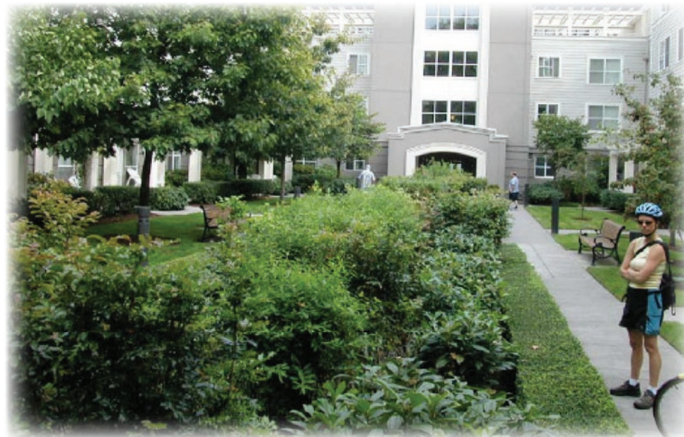
INFILTRATION PLANTER- USE WHEN YOU WANT THE WATER TO PERCOLATE INTO THE GROUND.
