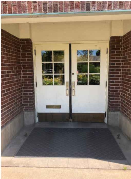
Exterior doors and hardware, not original
