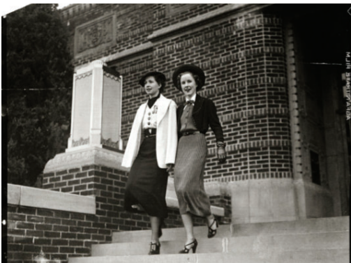
North entry steps, c1940
