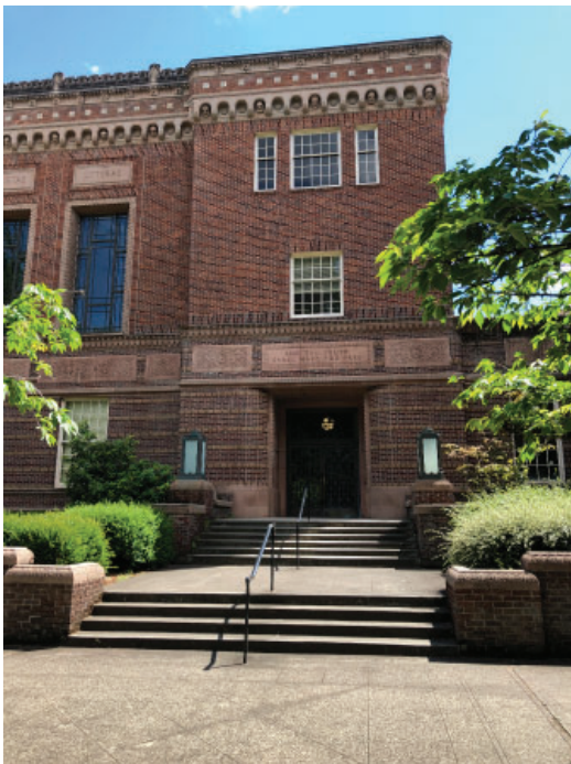
Exterior stair handrail, not original
