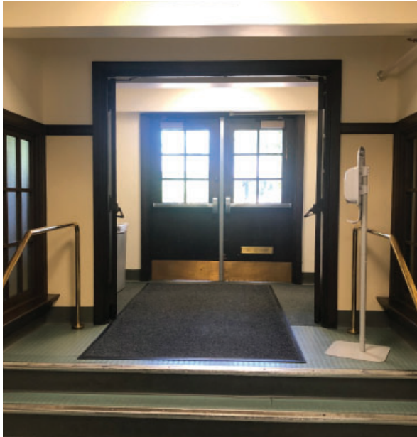
Basement hallway H002, wood doors, trim, and windows
