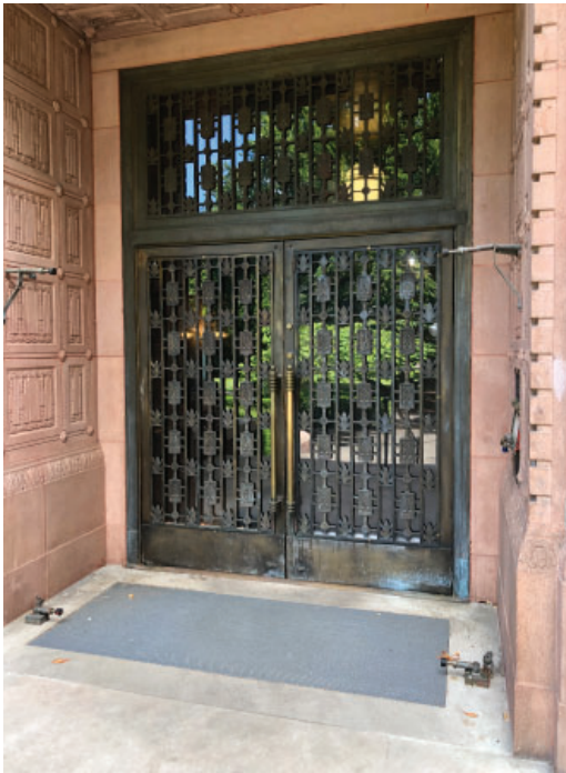
Decorative door pull finials (rods are not original). Exterior door fire egress hardware, not original
