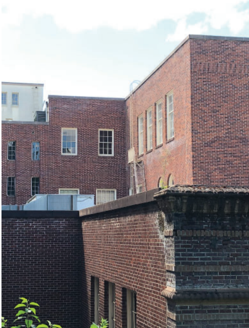
Roof ladder, not original
