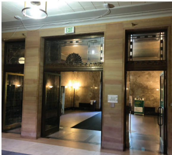
Entry lobbies L108 & L102, decorative interior details at both entries
