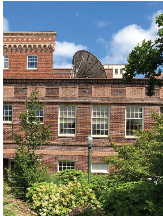
Satellite dish on roof, not original
