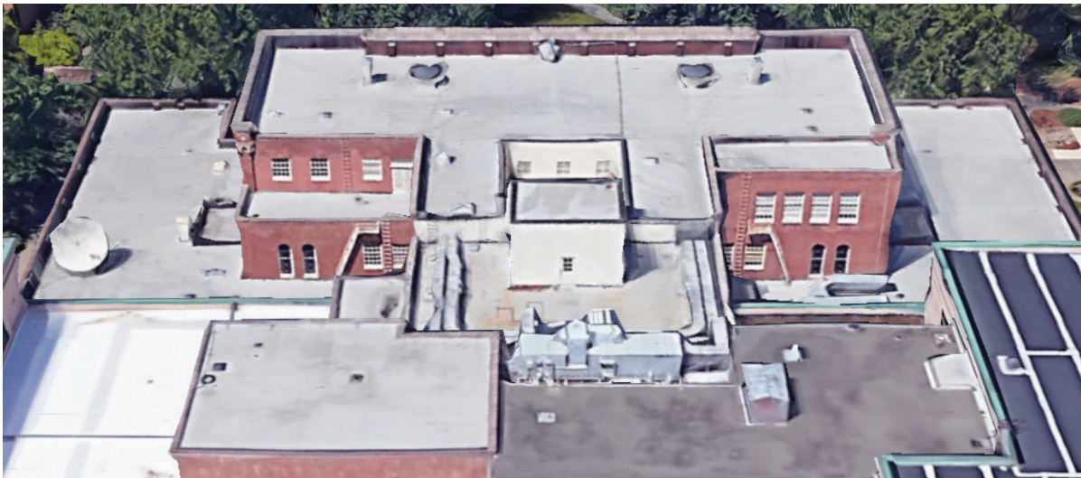
Existing South Elevation (1937 portion of building), Google Earth, 2022
