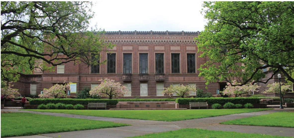
Existing North Elevation, 2022
