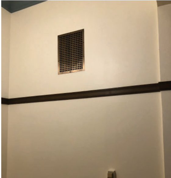
1st floor hallway 101, metal vent cover, wood wall trim
