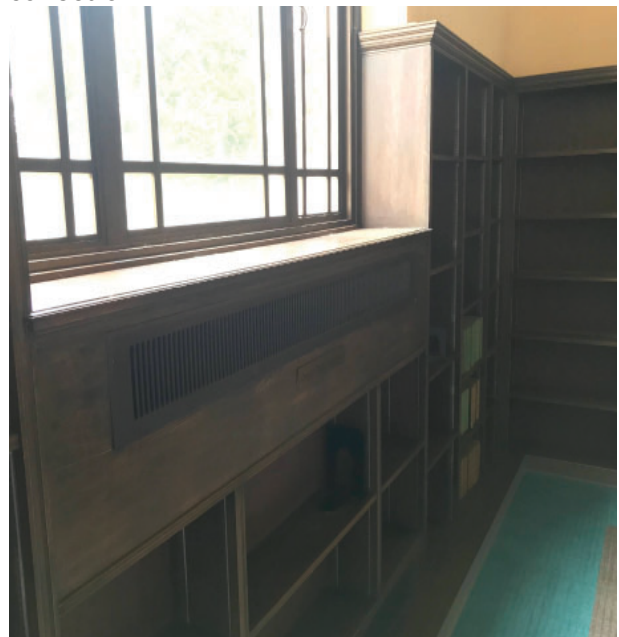
Room 206, Special Collections, wood built-ins and window trim, HVAC vent cover
