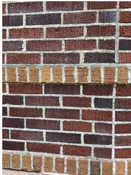
Visible differences in brick and mortar repairs
