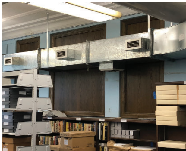
Room 301, covered windows (not original)
