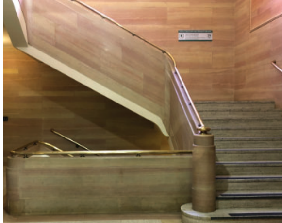
All floors stairwell, marble walls and balustrade
