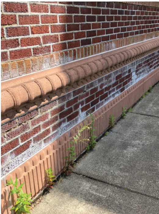
Brick efflorescence
