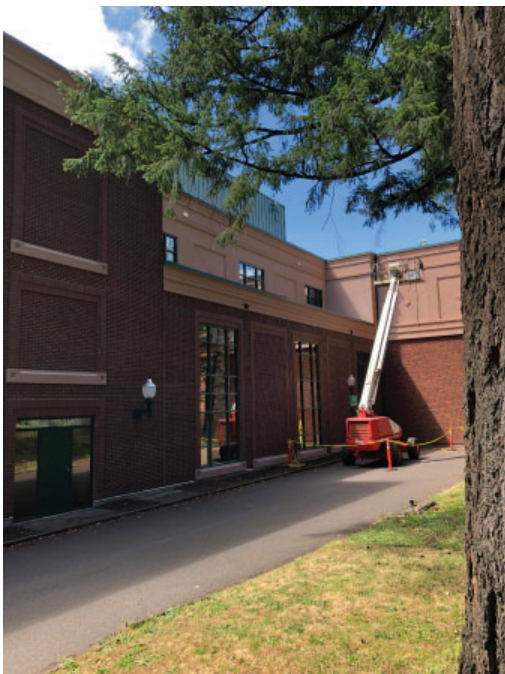
1966 and 1994 south library additions, not original (southeast corner)
