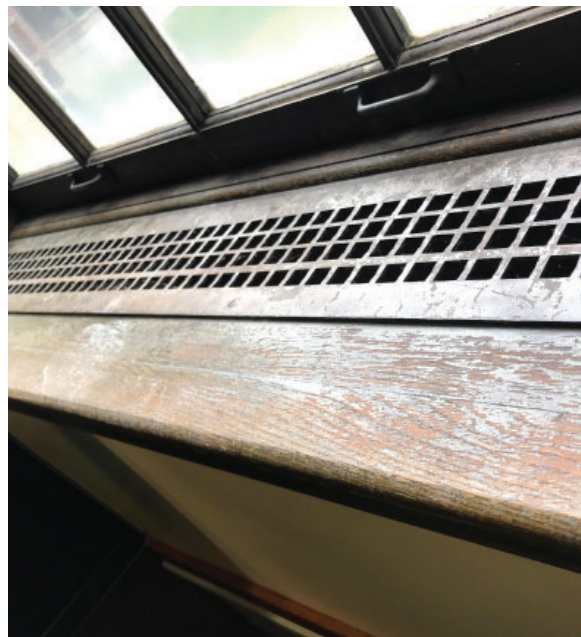
Room 115H, metal vent cover and window hardware
