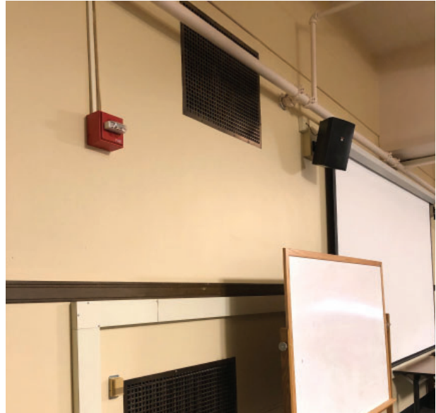
Room 101, metal vent cover
