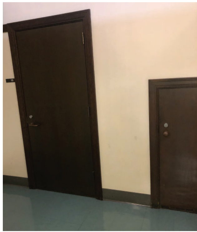
Basement hallway H010, under stair wood storage doors
