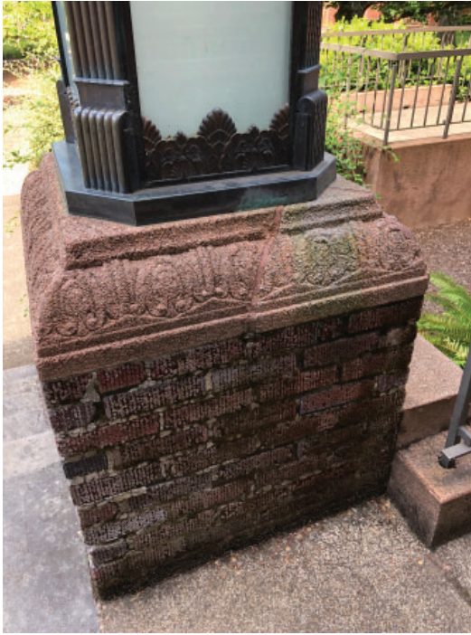
Visible repair in stone and brick
