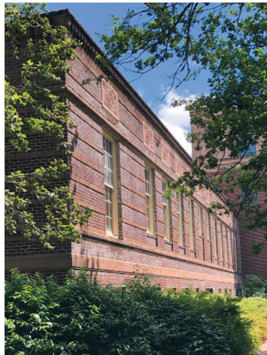
Biological growth on brick facade
