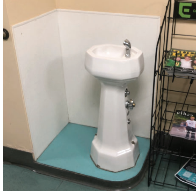
Basement hallway H002, drinking fountain
