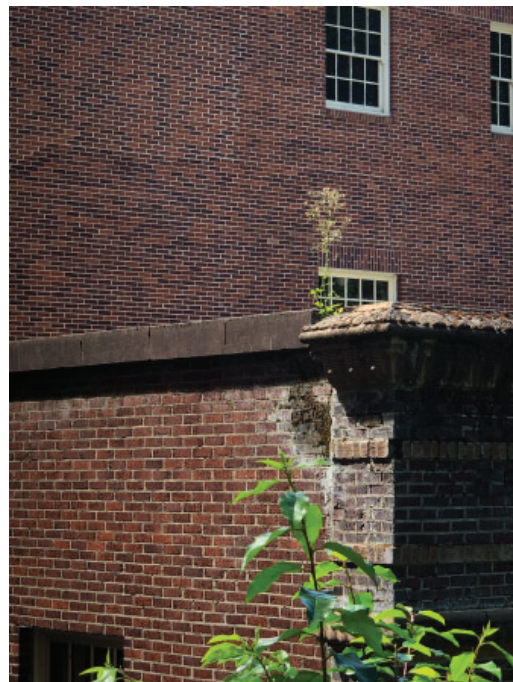
Biological growth on brick and stone; staining
