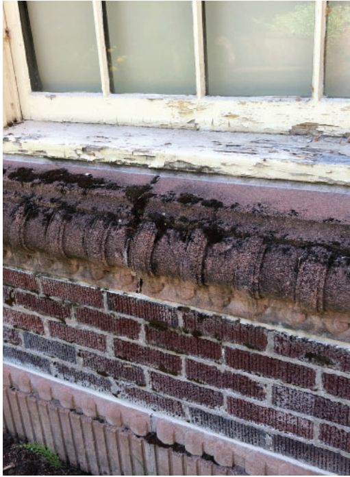
Painted wood windows showing signs of weathering Biological growth on stone and brick
