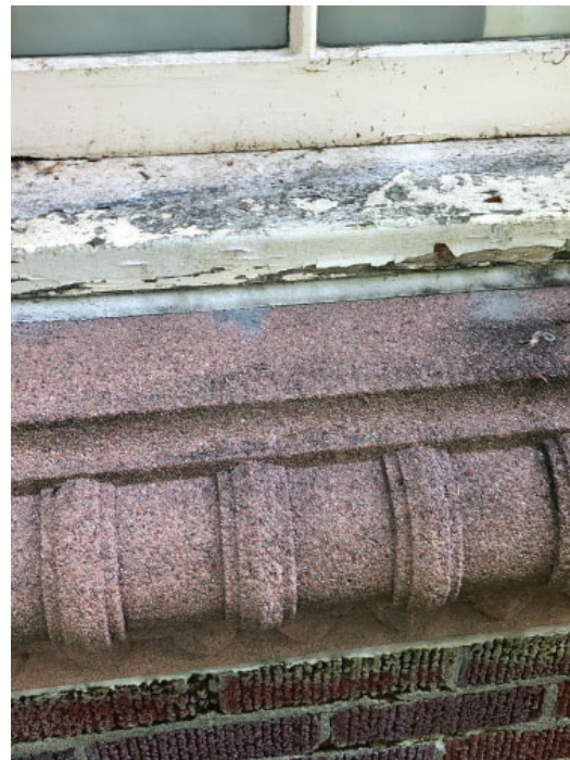
Painted wood windows showing signs of weathering
