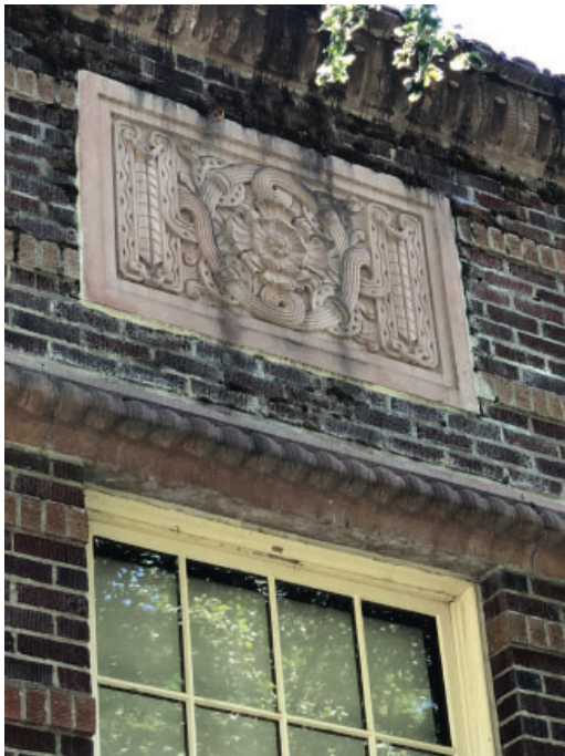
Biological growth on brick and stone; staining
