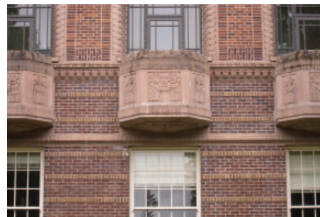
6. Facade: Exterior ornamentation (flame & cross on balconies)
