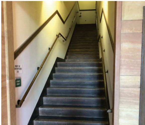
Stair S207 & S203, wood chair rail trim
