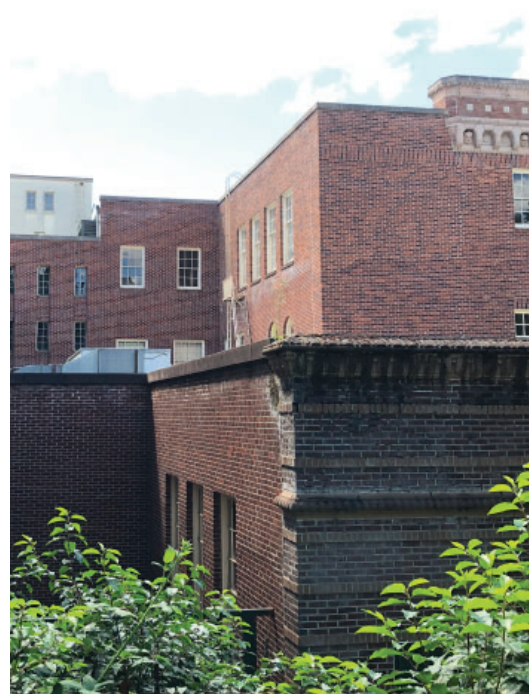
HVAC installed on roof, not original Biological growth on brick and stone
