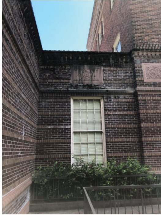
Biological growth on brick and stone; staining
