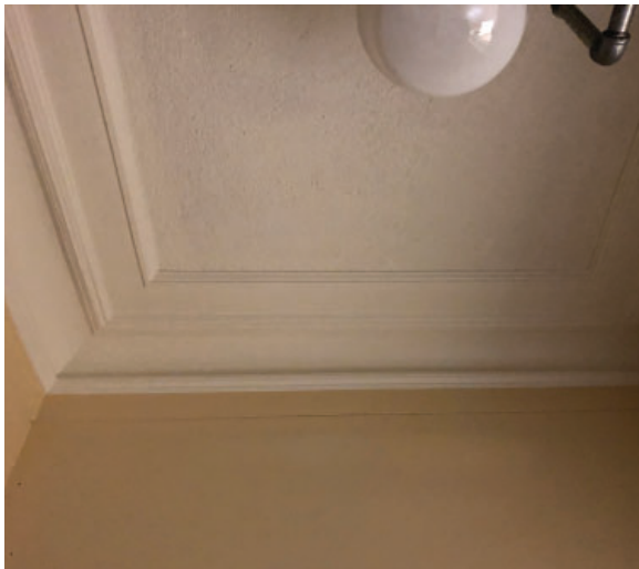
Room 301, ceiling crown molding
