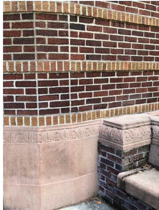
Differences in joint compound, showing repairs
