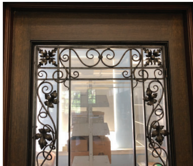
Room 301A, decorative door details
