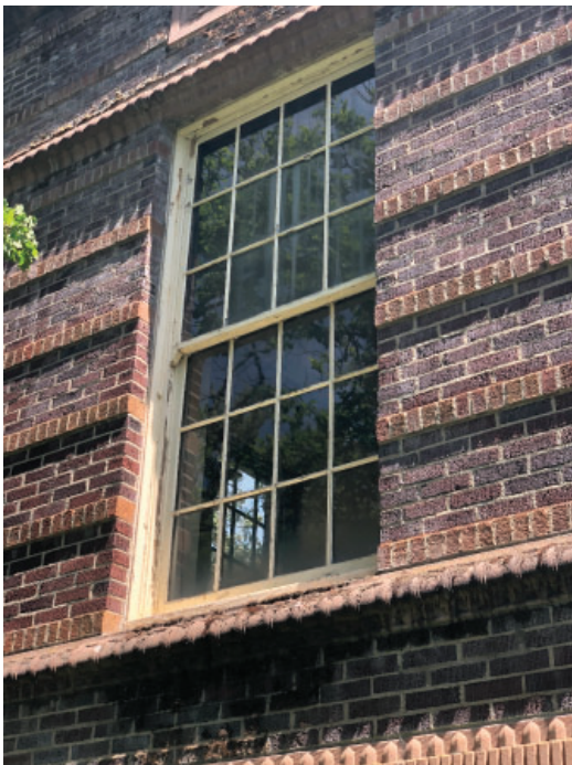
Painted wood windows showing signs of weathering
