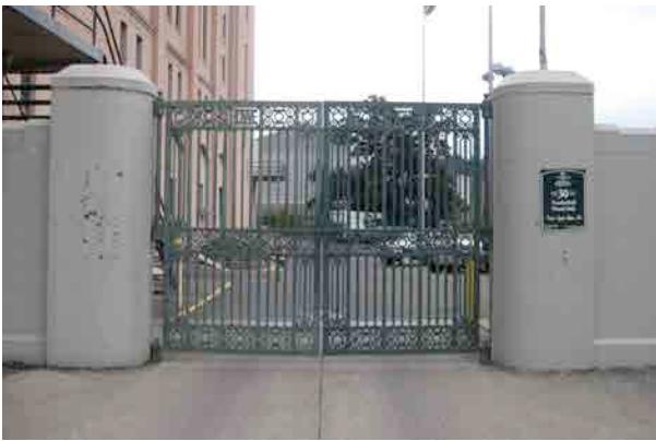
Main Howe Gates and concrete wall, Looking East
