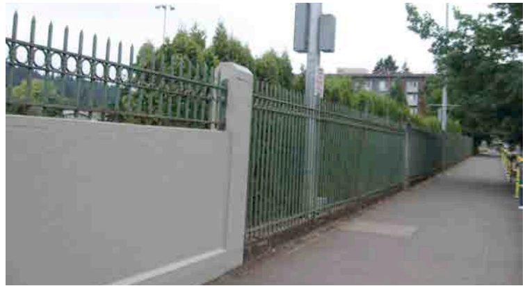
Concrete Wall and Wrought Iron Fence
