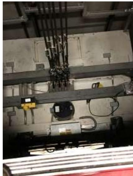
Fig. 8 – Elevator car top
