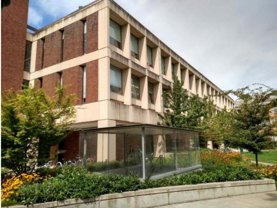
Photo 1 – End Wall w/ Discontinuous Lateral Elements and Unanchored Brick Veneer
