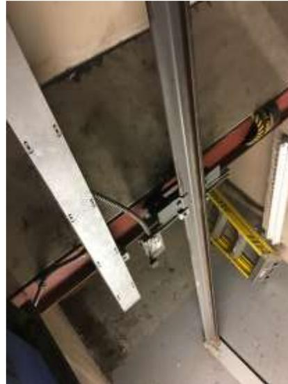
Fig. 4 – Divider beam (red) that can be relocated to the north by 8" to 10".
