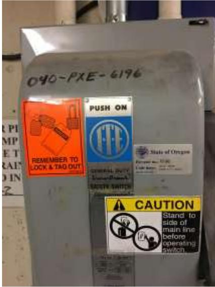
Fig. 5 – Three phase disconnect mounted on hinge side of the door.
