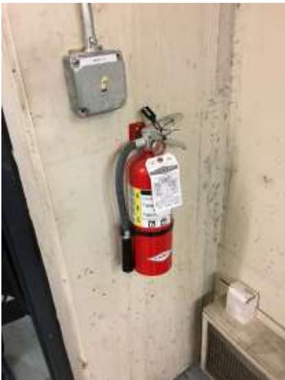
Fig. 3 – Fire extinguisher mounted near door.
