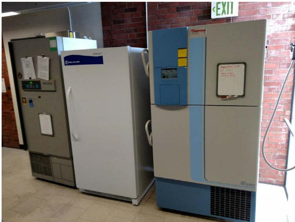
Photo 6 – Unbraced Equipment Adjacent to Exit
