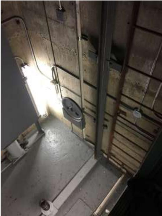
Fig. 14 – The hoistway is 6'-1" deep at the machine pedestal and 7'-1" at the counter weights. The current width is 8'-7 ¼" to divider steel. Relocating the divider steel can achieve additional 10" in width.
