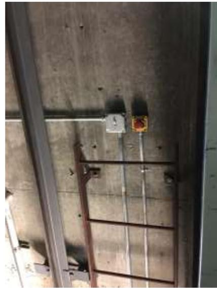
Fig. 10 – Pit ladder needs to be altered to current code – 48” above sill. 12” wide and a minimum of 4.5” from wall.
