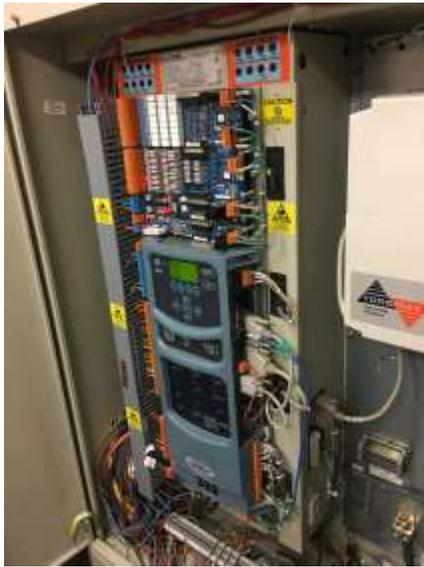
Fig. 9 – Current MCE controller with MAXTORQ drive. Replaced in 2008.
