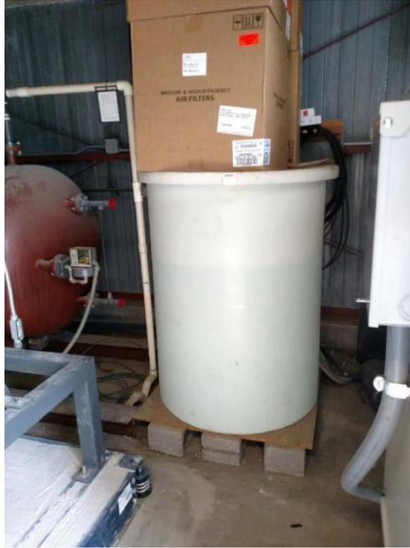
Photo 5 – Unbraced Tank In Mechanical Penthouse
