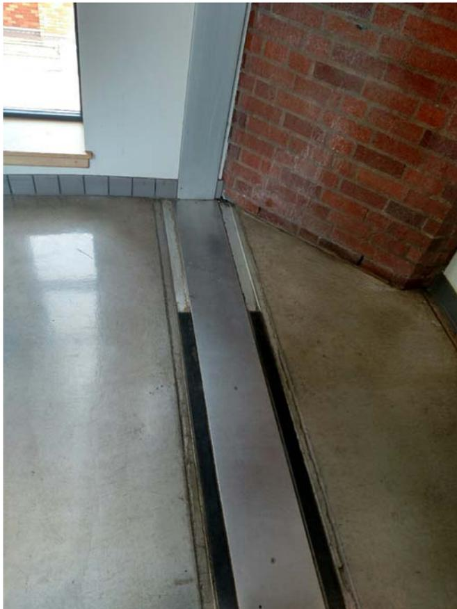
Photo 2 – Seismic Joint at Streisinger Hall
