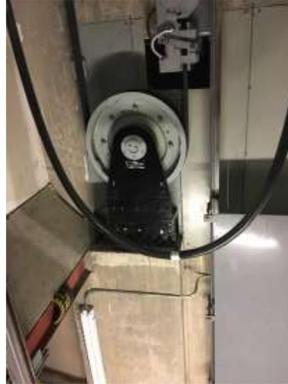
Fig. 2 – Governor tail sheave was replaced in 2008
