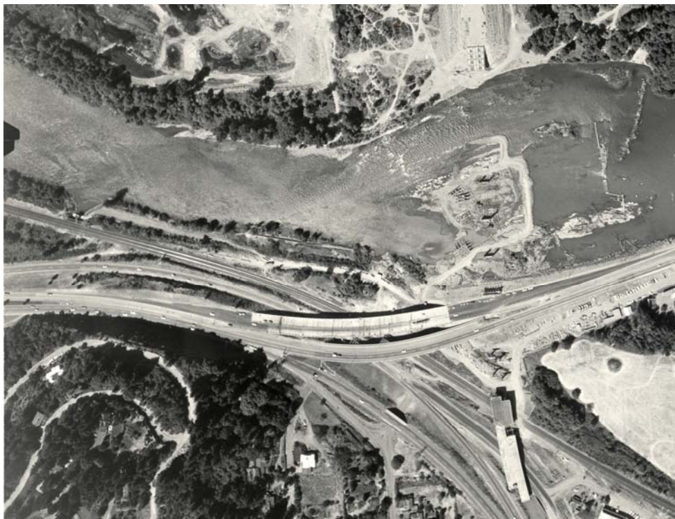
Figure 4. Aerial photograph taken in 1960 showing bridge construction activities in the millrace area, as well as intake relocation and pump house near railroad overpass (ODOT JP8-5-60).
