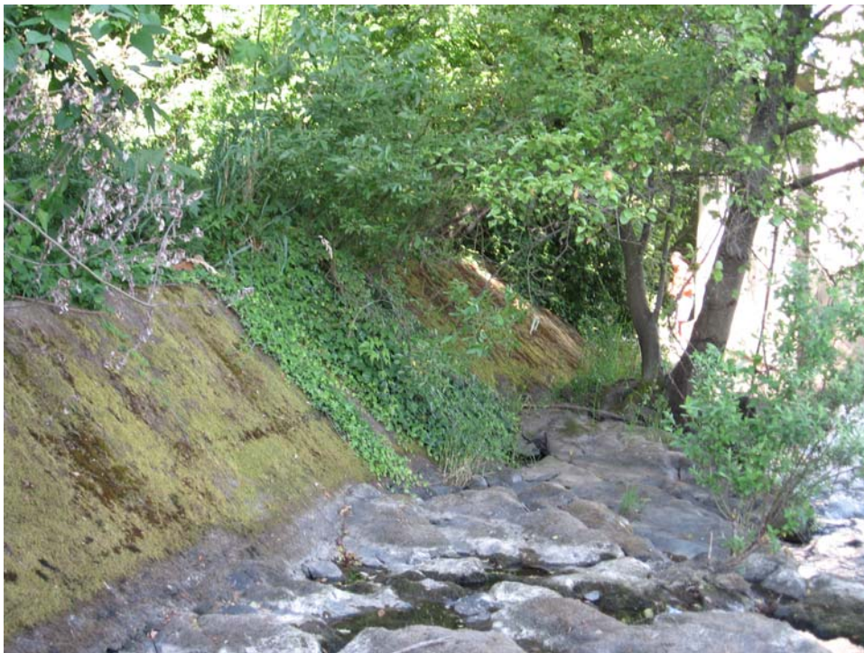
Figure 9. View to northeast of revetment from west side of detour bridge.
