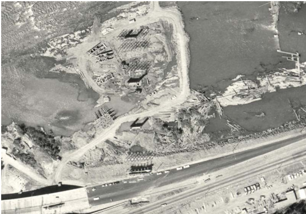
Figure 13. Enlargement of 1960 aerial photograph showing avoidance of millrace intake features within the I-5 construction corridor and the breaching of the millrace revetments to the west to allow construction access (ODOT JP8-5-60).
