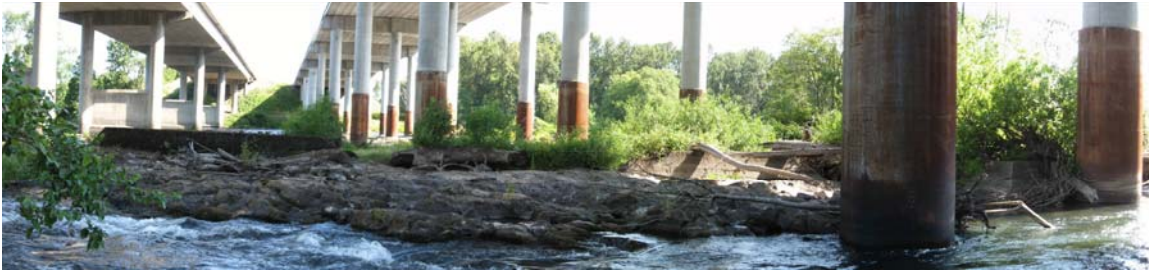
Figure 6. View to north from south shore of revetments and features associated with the intake gate (#5) and log crib (#4) beneath original I-5 bridge (left) and detour bridge (right).
