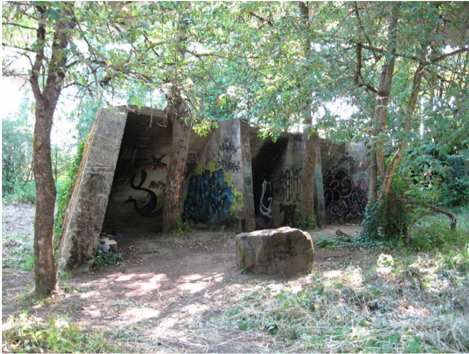
Figure 8. Reverse view of revetment shown in Figure 7 with I-5 bridge visible in upper corner.
