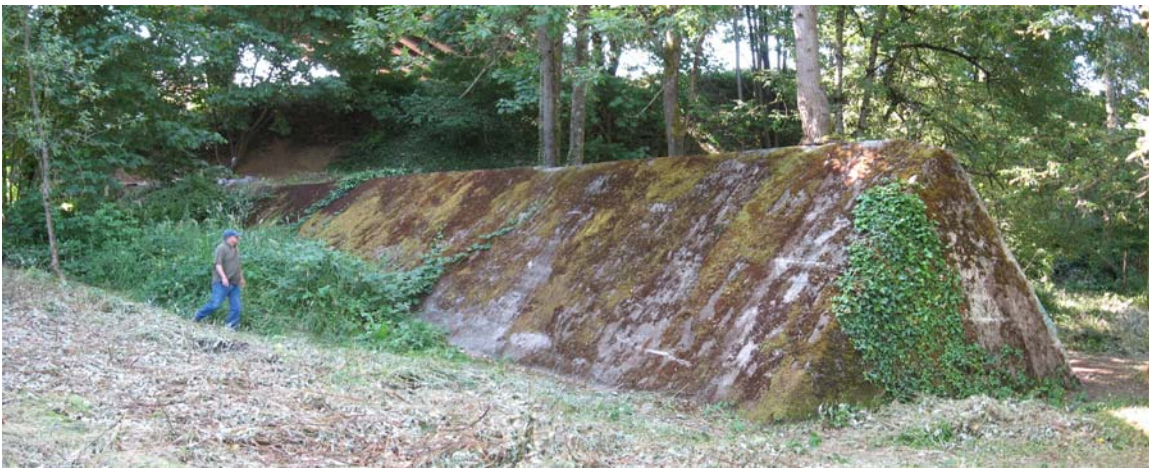
Figure 7. View to southeast looking toward the original I-5 bridge (in background) showing large revetment marking former millrace channel.
