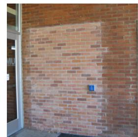
Opening infilled in 1998; new doors to the left installed.
