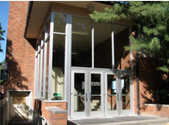
South Entrance aluminum storefront system replaced in kind in 2009. Original 1962 brick & limestone walls
