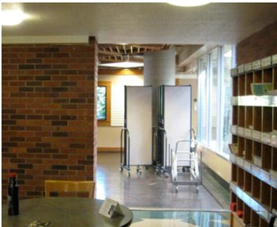
One of three openings in lobby cut in original exterior wall to make way for 1973 skybridge.
