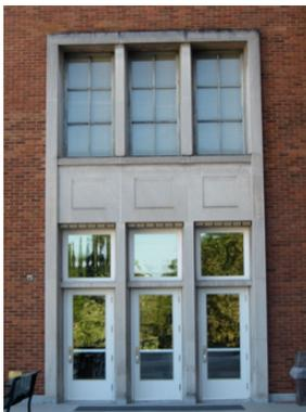
(1) Replacement doors & hardware in 2009. Original cast concrete detailing & upper level windows.
