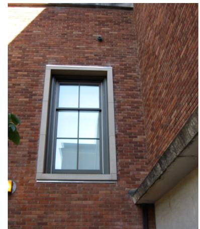
New opening for a window cut in south-facing wall to match existing during 2007 remodel.
