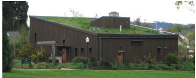
Many Nations Longhouse bioswale and green roof
