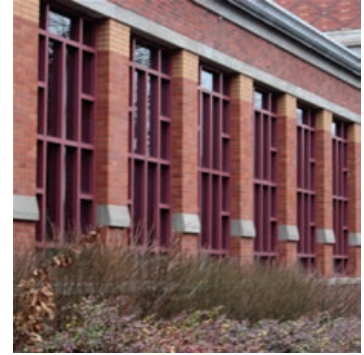
Rhythm of Windows - Repetition of windows break up the scale of the facade (e.g., openings separated by columns or other vertical elements or recessed windows). As a general (but not absolute) rule, avoid large, blank facades, large areas of glazing, or unbroken, horizontally oriented windows (ribbon windows).
