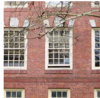
Rhythm of Windows - Repetition of windows break up the scale of the facade (e.g., openings separated by columns or other vertical elements or recessed windows). As a general (but not absolute) rule, avoid large, blank facades, large areas of glazing, or unbroken, horizontally oriented windows (ribbon windows).
