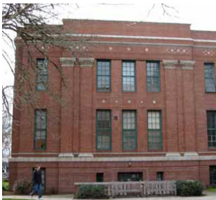
Composition - Buildings should be vertically composed of three parts: top, middle, and bottom. Provide distinction through the use of horizontal lines, such as banding, use of different materials, or variation in patterns and textures.
