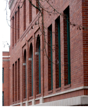
Rhythm of Windows - Repetition of windows break up the scale of the facade (e.g., openings separated by columns or other vertical elements or recessed windows). As a general (but not absolute) rule, avoid large, blank facades, large areas of glazing, or unbroken, horizontally oriented windows (ribbon windows).
