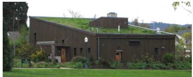
Many Nations Longhouse bioswale and green roof
