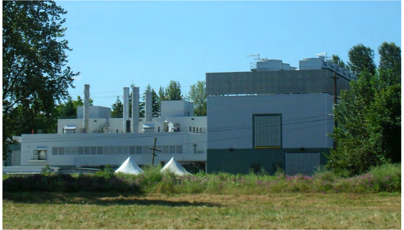
University of Oregon Power Plant viewed from the riverfront
