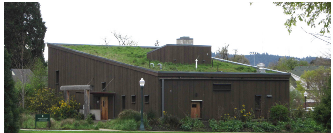
Many Nations Longhouse bioswale and green roof
