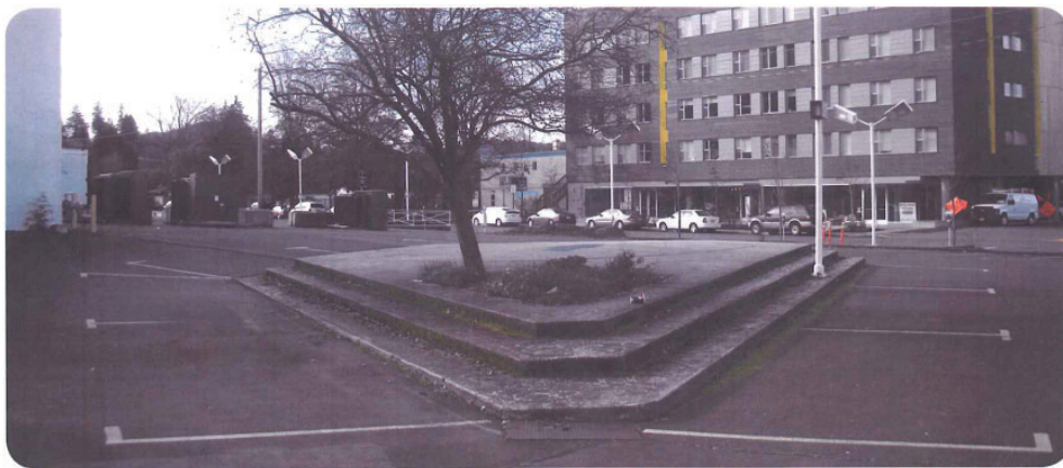
Figure 3.7: This raised concrete pad, a character-defining feature, originally was the slab for the Used Car Dealership Pavilion. It connected to the Showroom Pavilion via a causeway and was removed sometime after 1993. Source: Photograph by Author.
