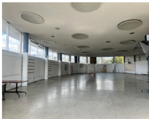
Original terrazzo floor in pavilion space; removal of office spaces from south wall
