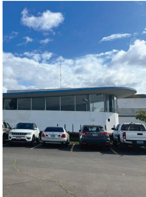
Post 2005 addition of plywood to showroom curtain wall
