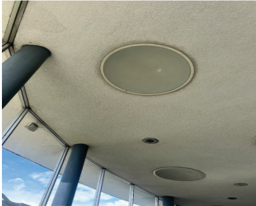
Original ceiling recessed light fixtures and original ceiling finish
