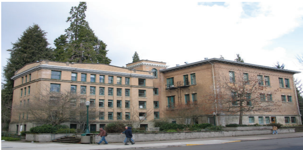
Figure 1. Fenton Hall, south elevation
