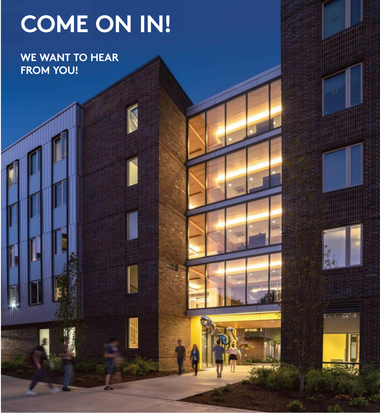
Residential Building C at Living Learning Center Green
