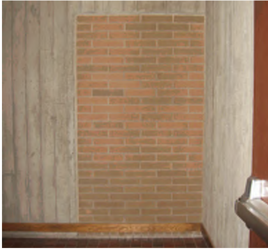
Stairwell 400 (Block out for future door; as seen on fourth floor floorplan)
