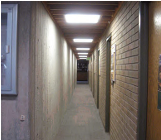
Hallway 301 (Wall material and suspended wood slat ceiling system)
