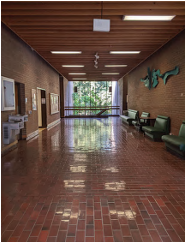
Hallway 225 (Flooring, suspended wood slat ceiling system, brick walls, window, and stairwell)
