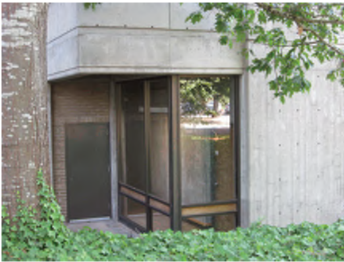
Windows with wood panel and concrete overhang.
