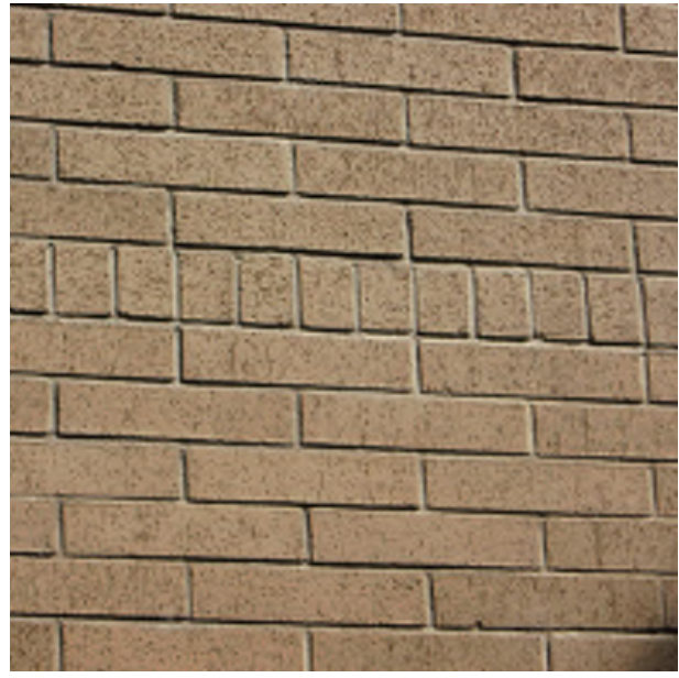
Change in brick orientation to signify floor divisions.
