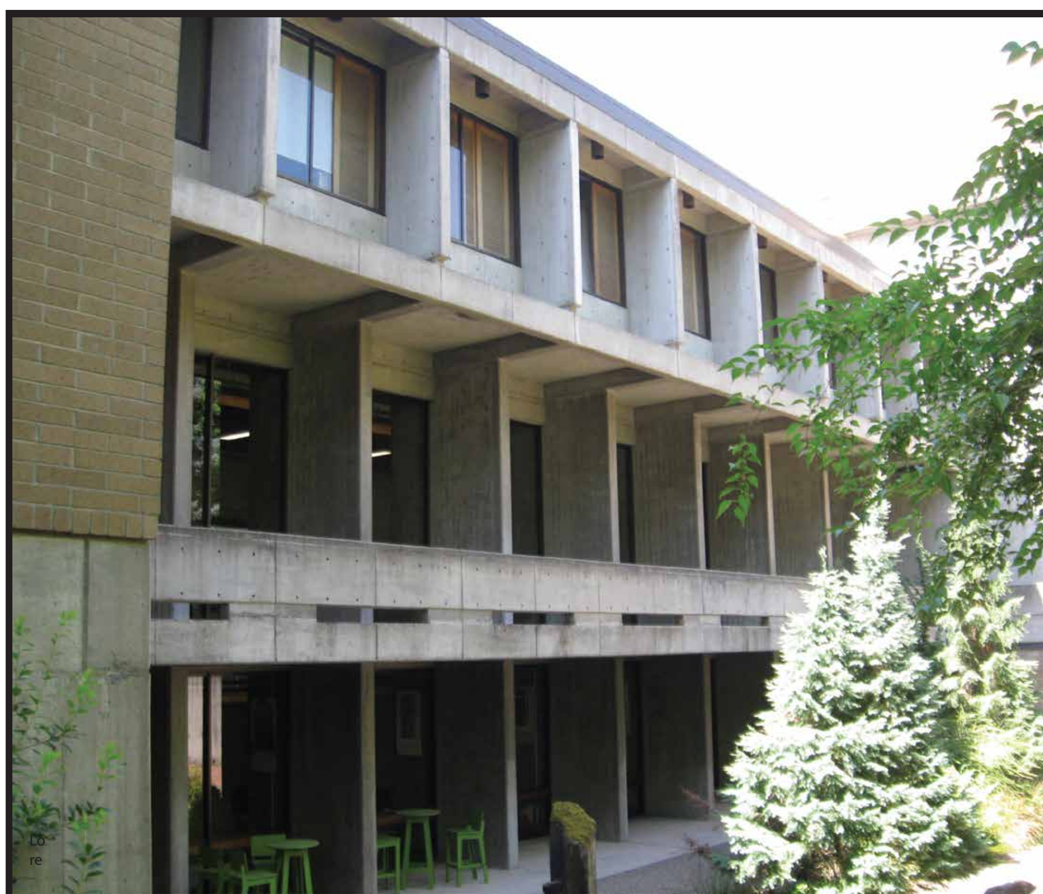
Geometric massings direct light from the West facade into the second floor hallways and third floor office spaces
