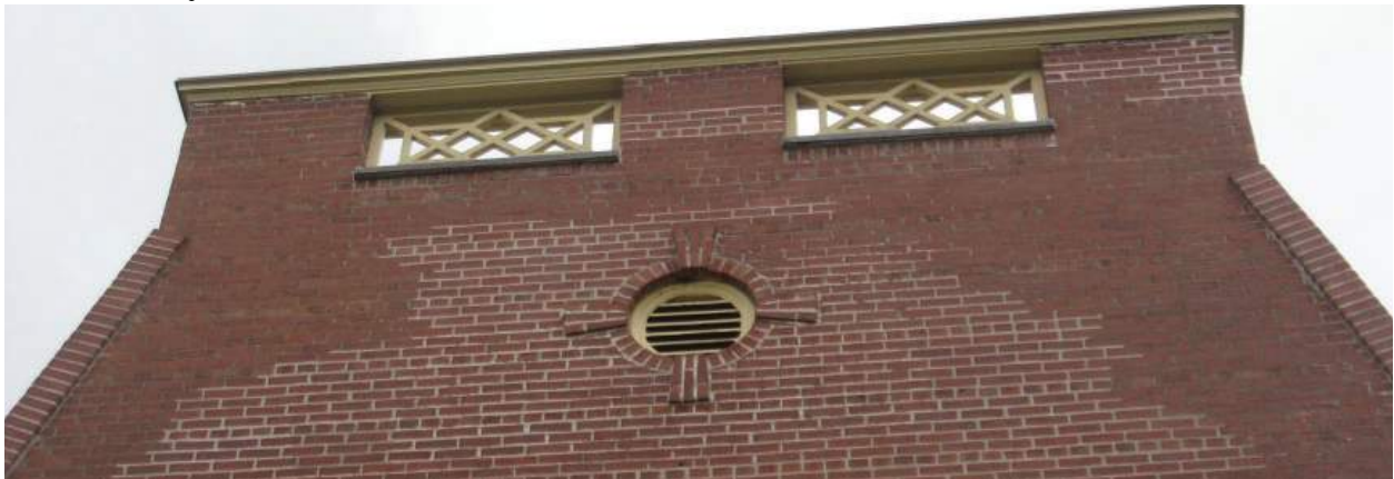
Parapets and oculus window, repointed brick and mortar. (West 2)
