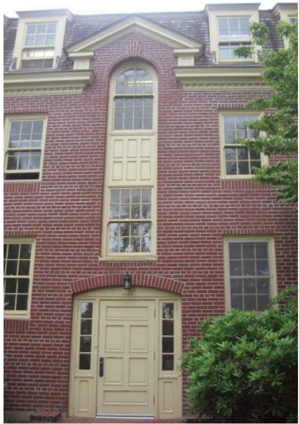
Door with jack arch and stacked windows. (North 3)
