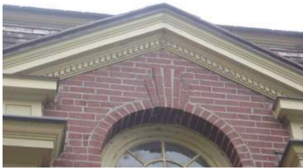
Cornice, jack arch, and pediment, restored cedar shingles on roof. (North 3)
