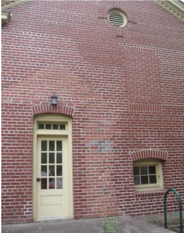
Window and awning removed, repointed brick and mortar. (East 1)
