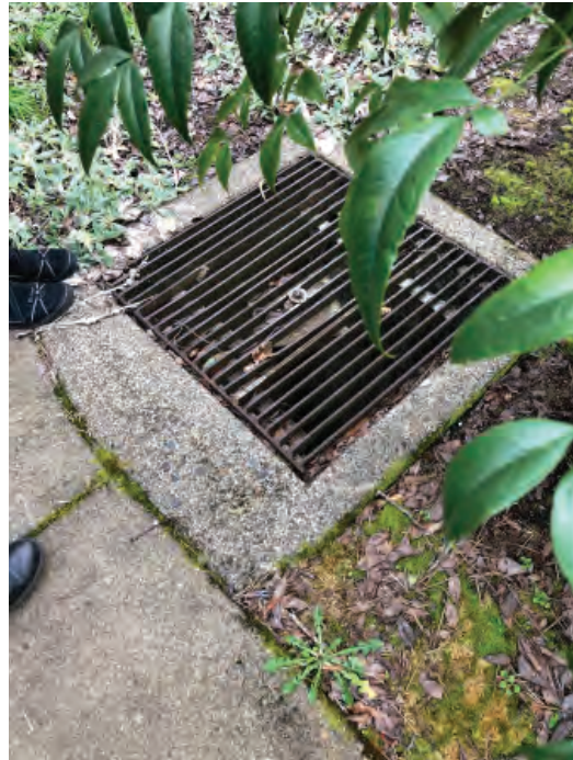
Storm drain inlet location in landscape, not original.
