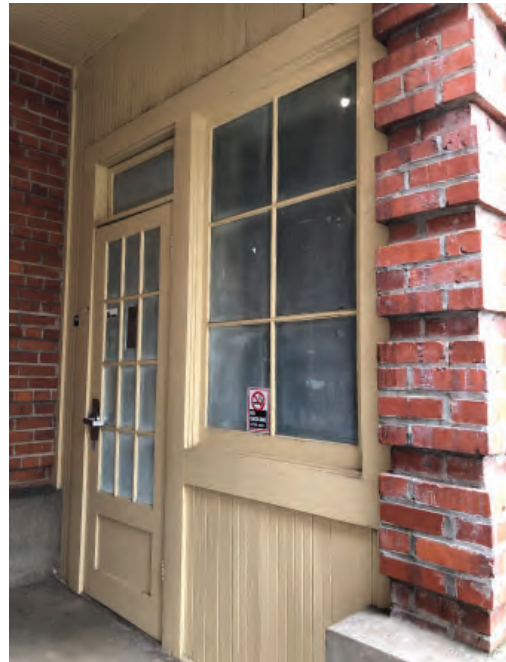
Original doors and windows.
