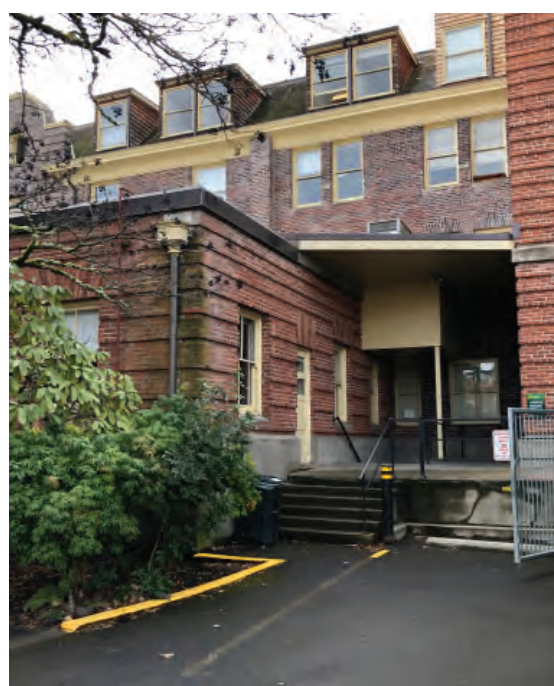
Dormers added to east facade. Overhang above the stairs and entrance is not original.
