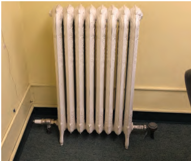
Room 308 (Ornamented Radiator)
