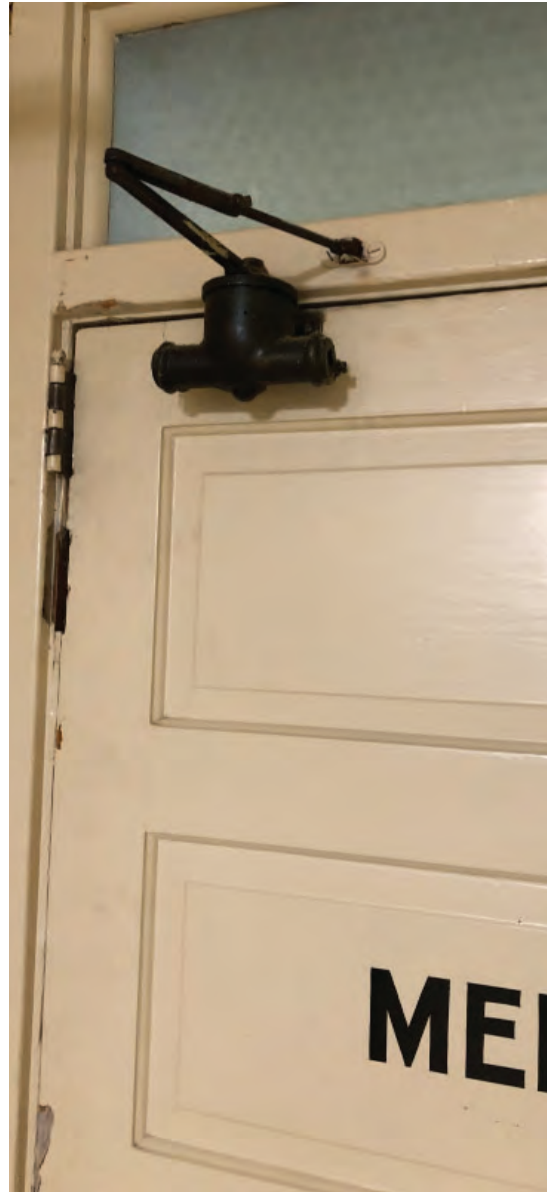
Mens Restroom (Old Hardware)
