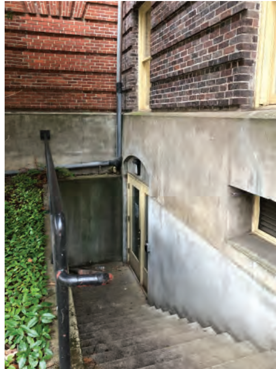
Stairwell leading down to basement shows foundation differences. Brick color differences between additions and original building.
