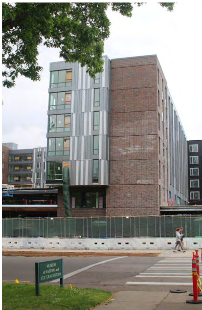
DeNorval Unthank Jr. Residence Hall Construction, 2021
