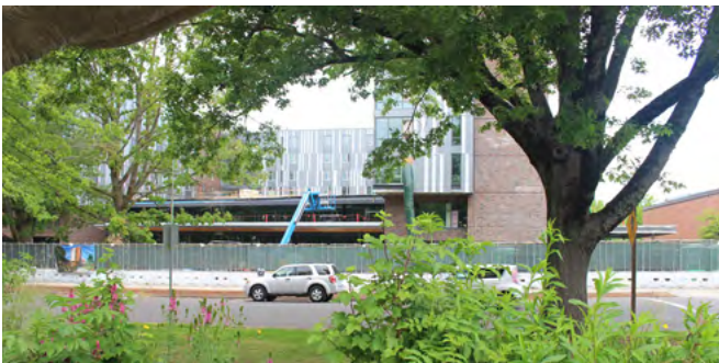
DeNorval Unthank Jr. Residence Hall Construction, 2021
