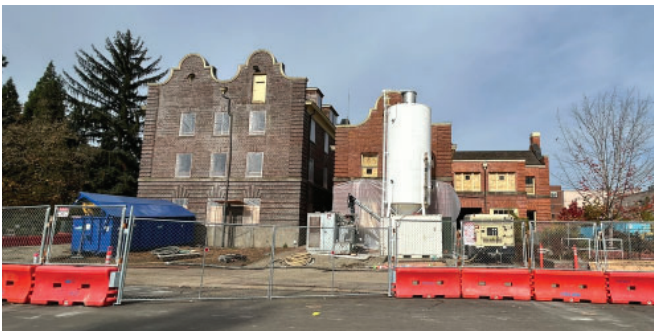
Friendly Hall Construction, 2025
