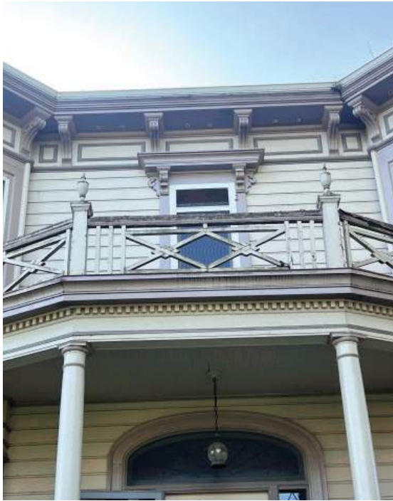
Second story balcony contains unoriginal wooden fretwork railing, balustrades, and finials; second story bracketed window crowns; decorative eave brackets
