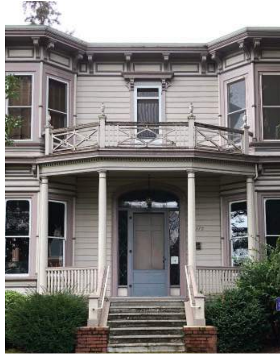
Symmetrical northern entrance with a central porch supported by round wood columns with capitals and entablature with dental course
