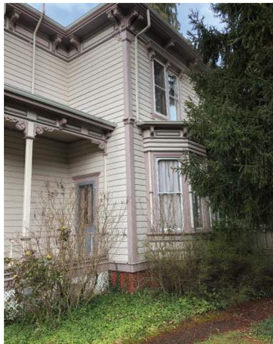
Original first floor bay window with wooden trim and moldings; decorative eave brackets, cornices, and frieze panels
