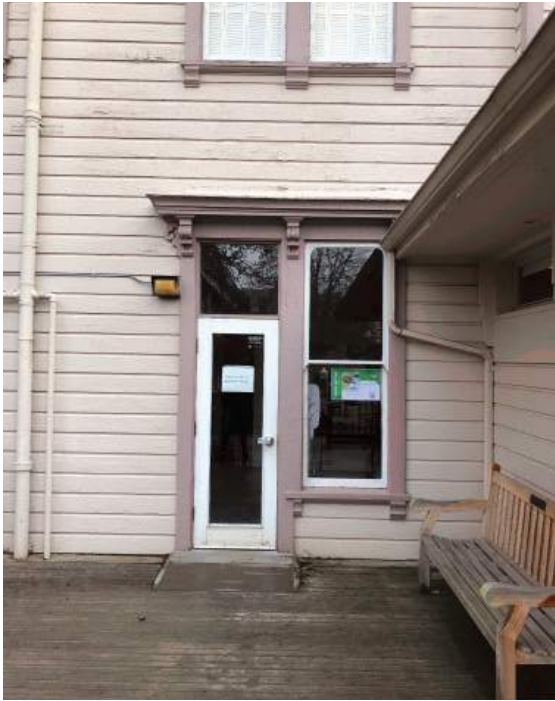
Window altered into door with single hung windows, incompatible light fixture, gutter downspouts
