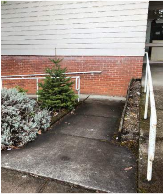
1963 addition with brick masonry foundation; exterior ramp and handrail
