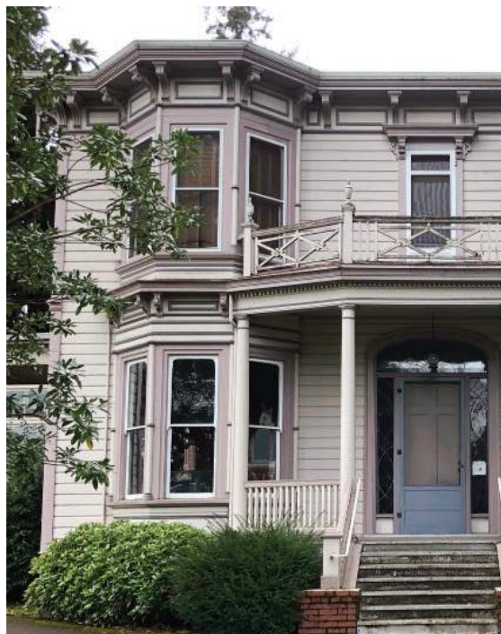
Original two story bay windows with three sided glass panes; cornices & frieze panels
