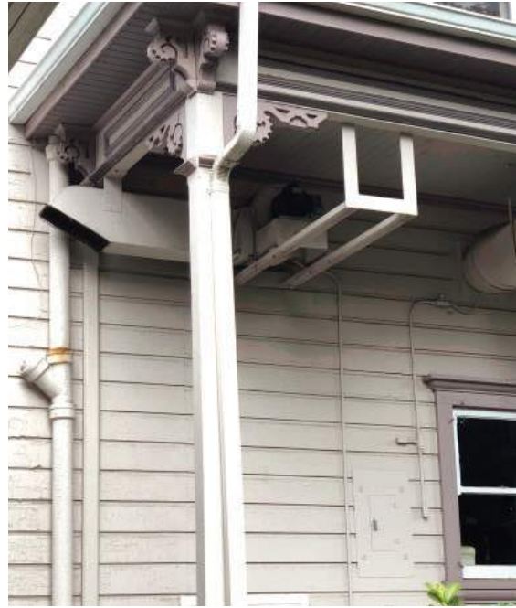
HVAC installed on east porch overhang; gutter downspout; electrical
