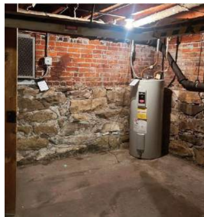
Heavy stone foundation; brick masonry walls
