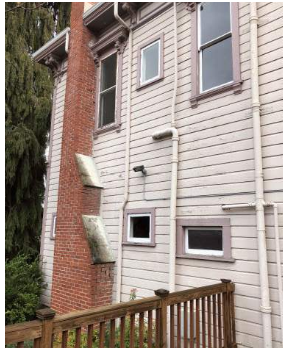
Brick chimney (1932), gutter downspouts, incompatible light fixture
