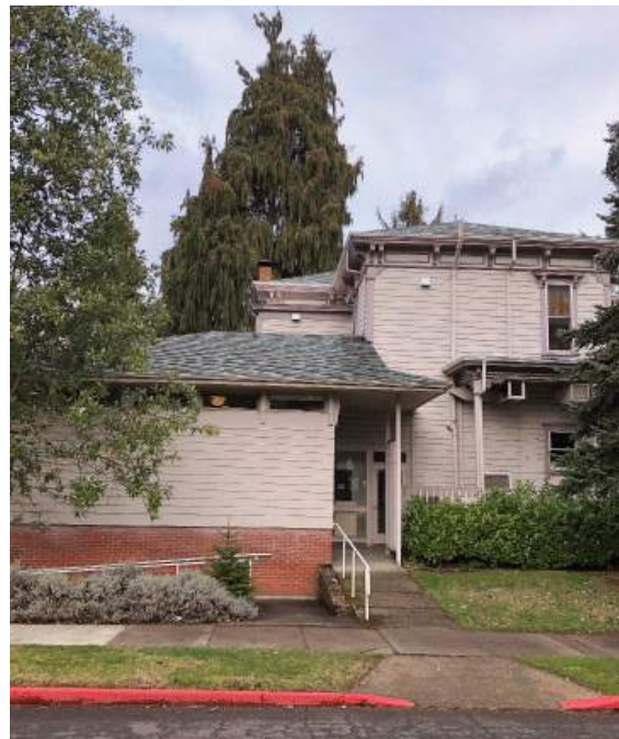
Wooden frame construction, brick foundation, and hip roof
