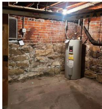
Heavy stone foundation; brick masonry walls
