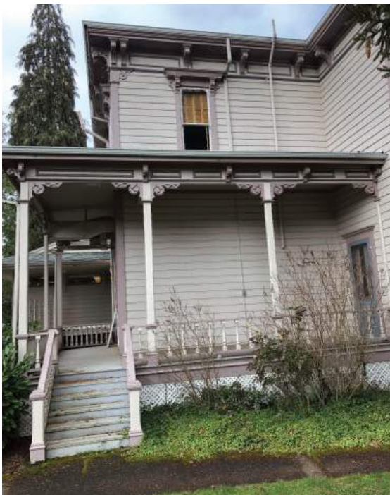
Decorative brackets support overhanging cornice below roof line
