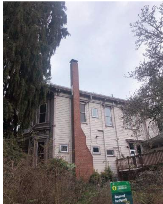
Brick chimney (1932), gutter downspouts, incompatible light fixture
