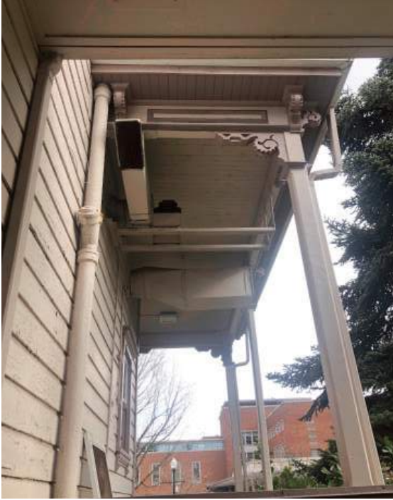
Incompatible light fixtures and HVAC equipment under porch overhang
