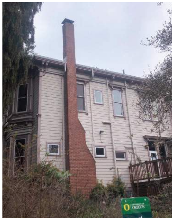
Wooden frame construction, brick foundation, and hip roof
