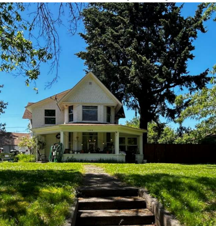
Photo: Historic Shoup House along Villard Avenue.
