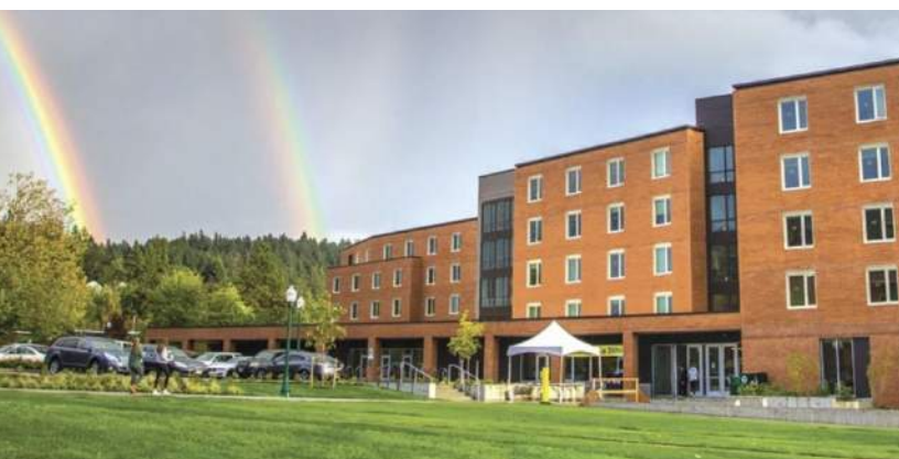
Photo: Kalapuya Ilihi Residence Hall.
