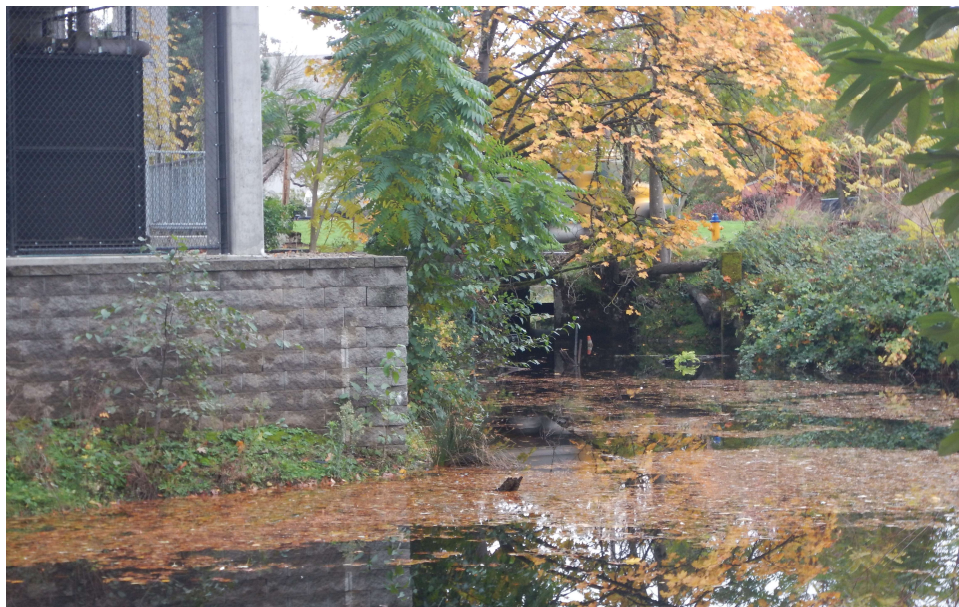
Figure 7. View looking through the Franklin culvert
