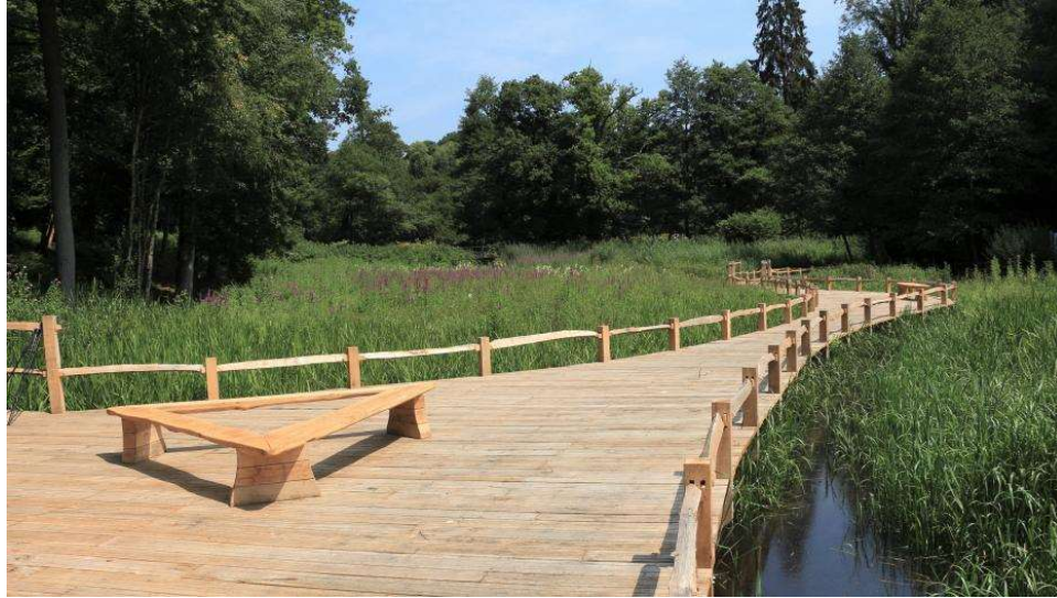
Figure 20. Targeted locations for boardwalks will allow visitors to more fully experience the wetlands
