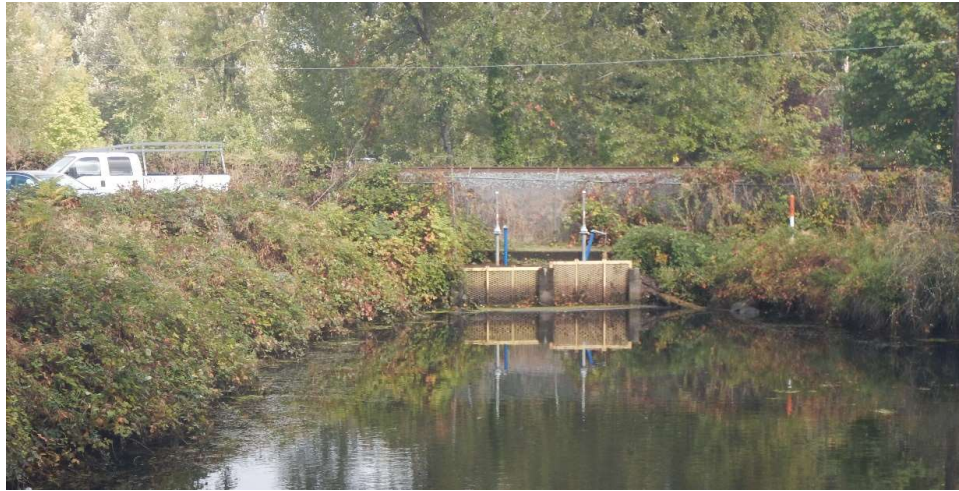
Figure 6. Water in the Millpond drains through this outlet structure to the north , to the Willamette River
