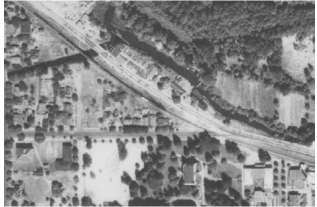
1936 Aerial Photograph showing houses and railroad still on site.
