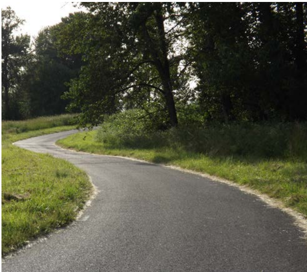
Primary pedestrian and bike path on site
