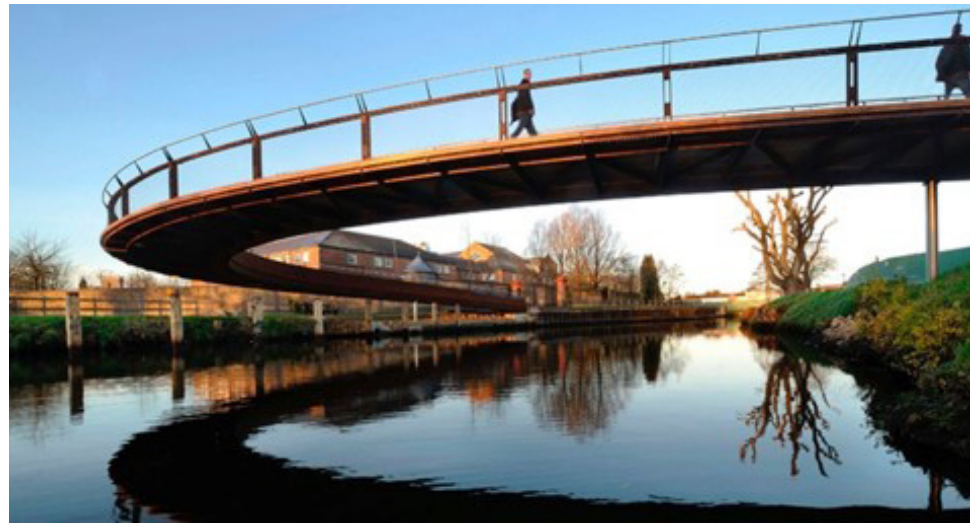
Jarrold Pedestrian Bridge, Norwich, UK
