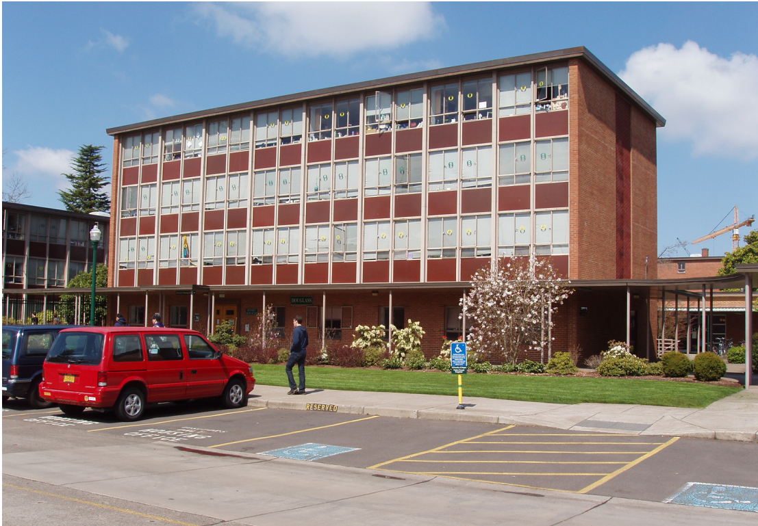
University of Oregon, Douglas Hall, Walton Housing Complex
