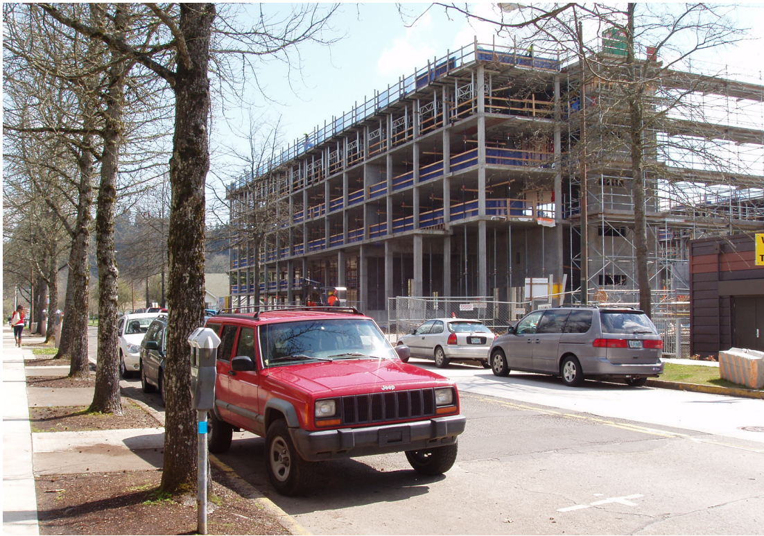
University of Oregon, East Campus Residence Hall, Under Construction
