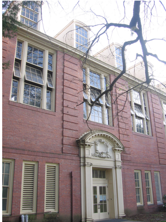
Figure 1. Gerlinger Hall, north elevation detail.
