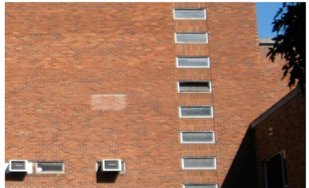
Infilled window on second floor at the time of 1985 addition of ballroom backstage.
